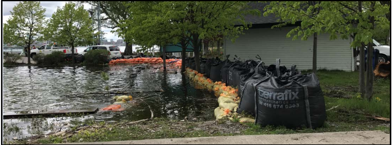
Figure 5-28: Sandbagging on Toronto Island, May 26, 2017. Photo credit: ©Toronto and Region Conservation (TRCA)
