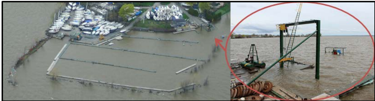
Figure 5-47: Beaconsfield Yacht Club showing inundation to a portion of the shoreline facilities on May 7, 2017. Photo credit: (left) Transport Canada - National Aerial Surveillance Program, (right) Jacob Bruxer, ECCC, May 5, 2017.
