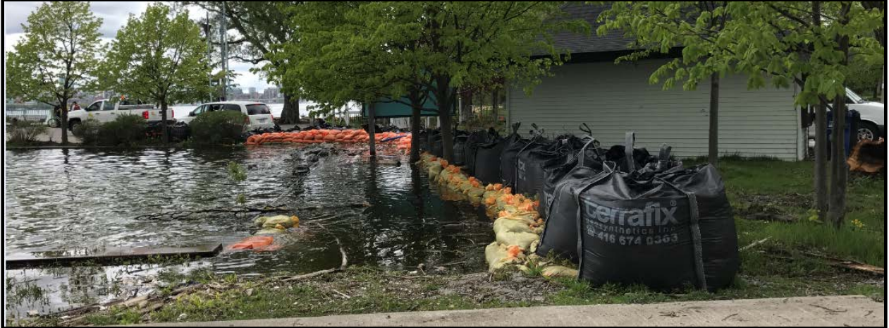
Figure 5-28: Sandbagging on Toronto Island, May 26, 2017. Photo credit: ©Toronto and Region Conservation (TRCA)
