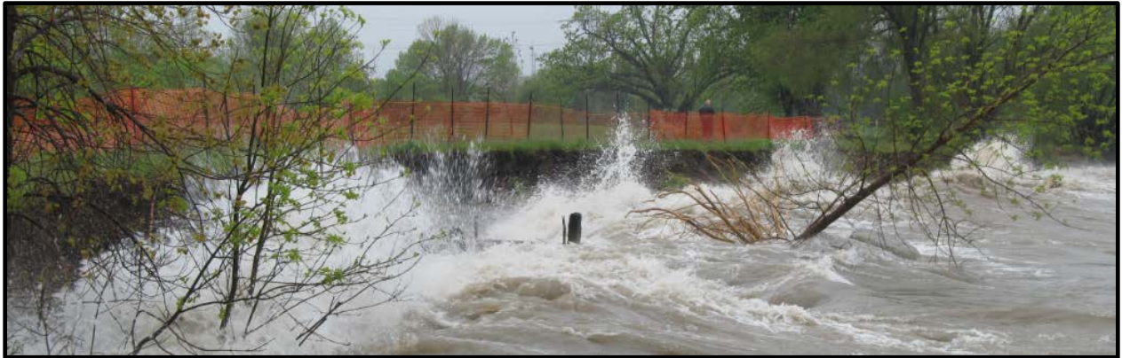
Figure 5-35: Shoreline erosion at Confederation Beach Park, City of Hamilton (photo taken May 17, 2017). Photo credit: City of Hamilton.
