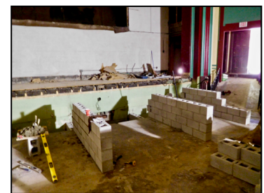
Stage under construction
