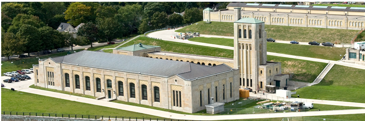
Figure 5-1: RC Harris Water Treatment Plant, Toronto, Ontario. Photo Credit: City of Toronto website: https://www.toronto.ca/services-payments/water-environment/tap-water-in-toronto/fast-facts-about-the-citys-water-treatment-plants/ .
