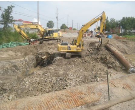
Dartnall Road Culvert
