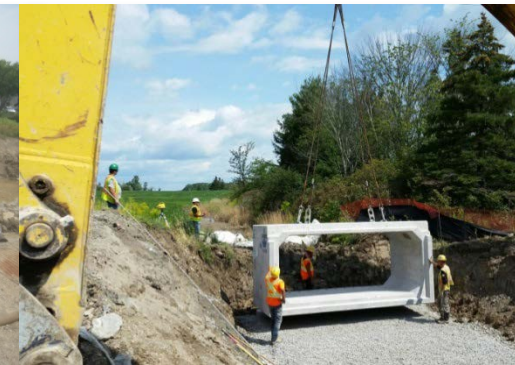
Bell Road Culvert Replacement
