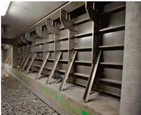
Myrtha Pools steel panel construction.
