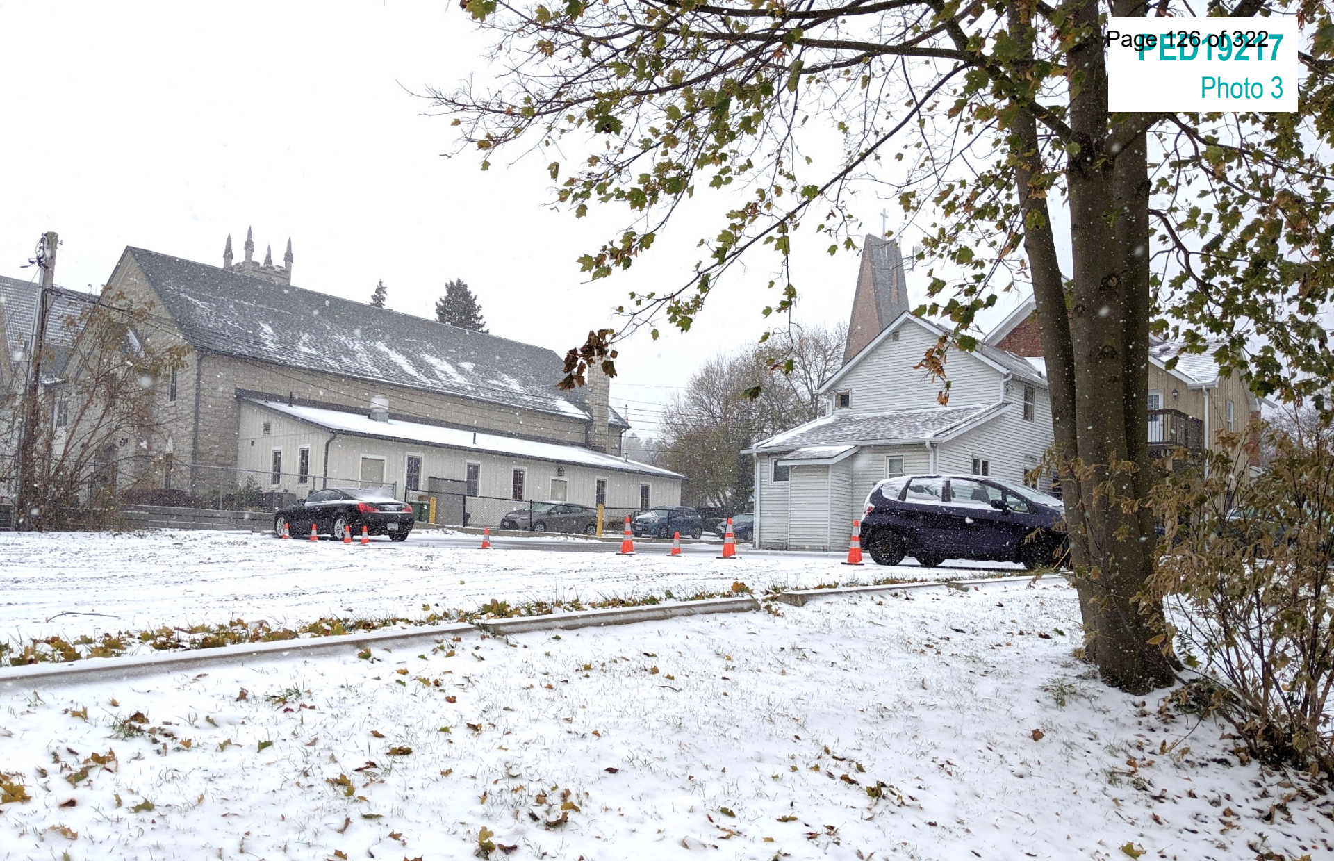
280 Wilson Street East from the rear, showing rear of existing building
