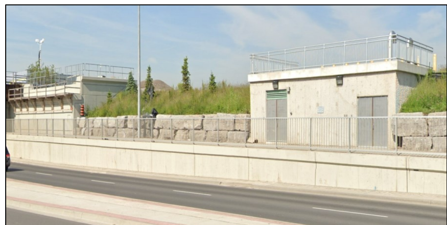
Centennial stormwater pumping station
