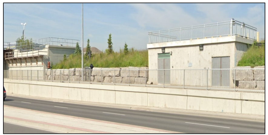
Centennial stormwater pumping station
