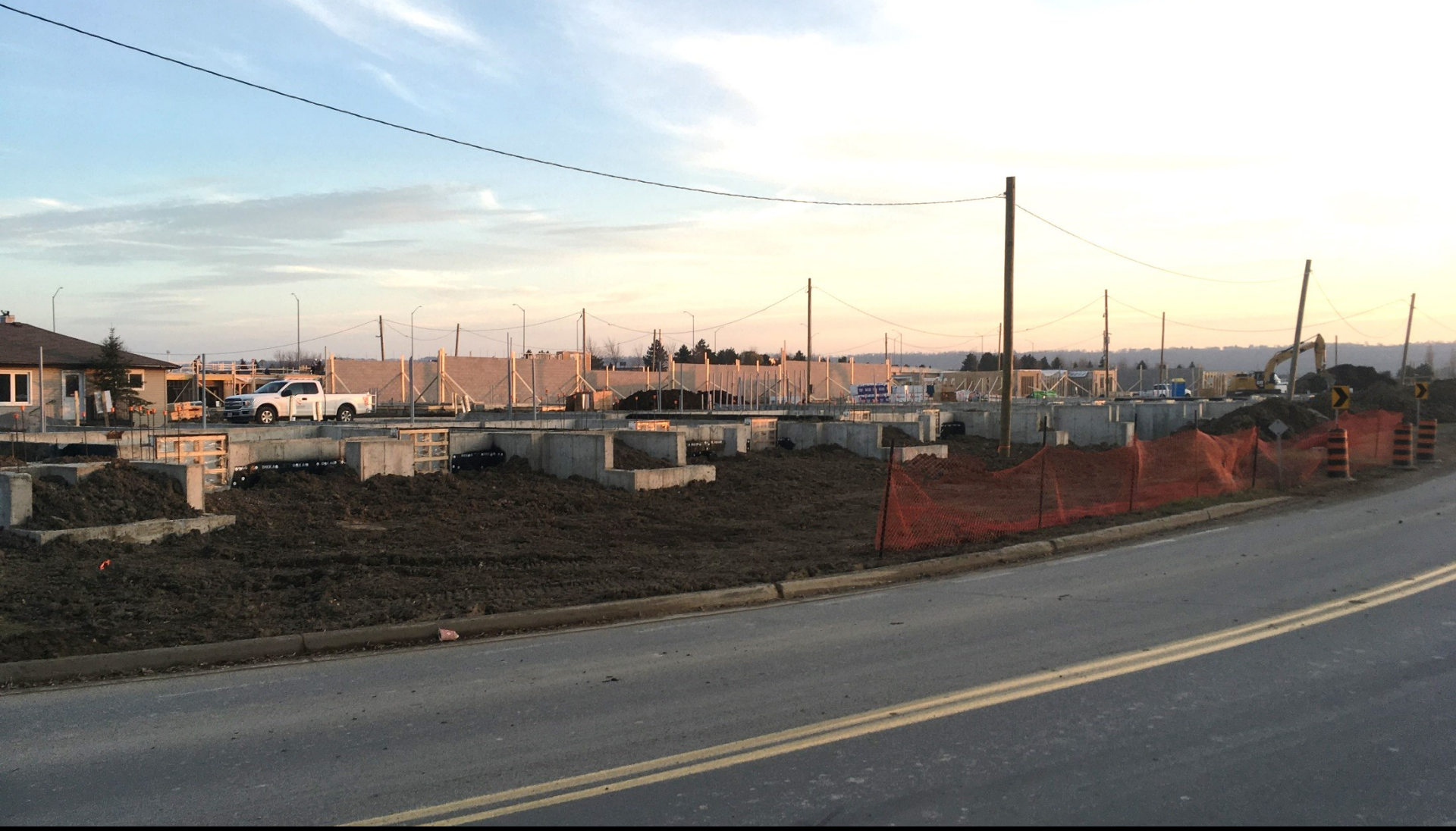
Looking south from where North Service Road turns into Lakeview Drive
