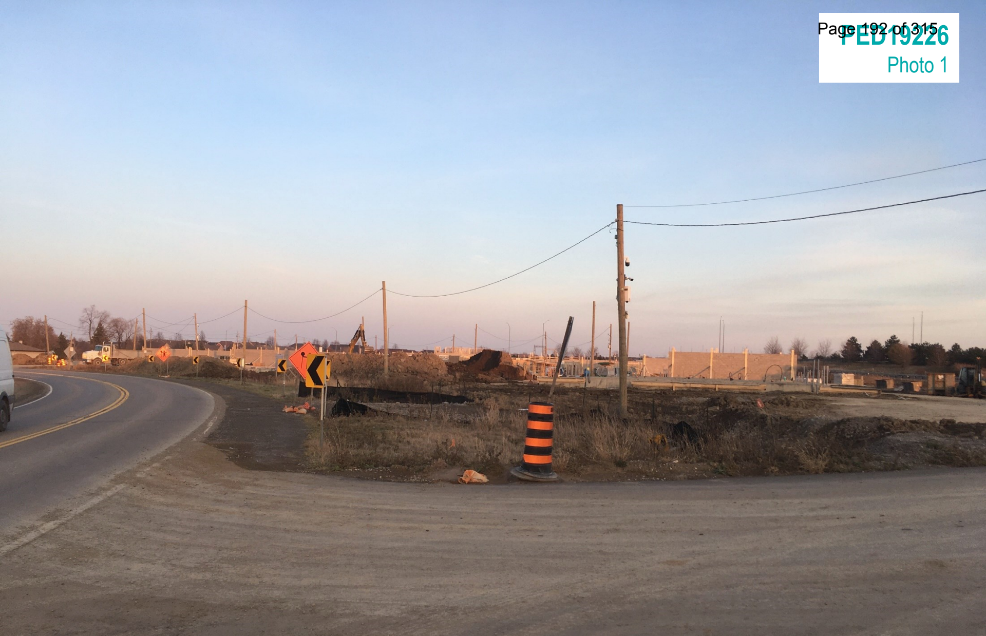
First entrance off North Service Road eastbound
