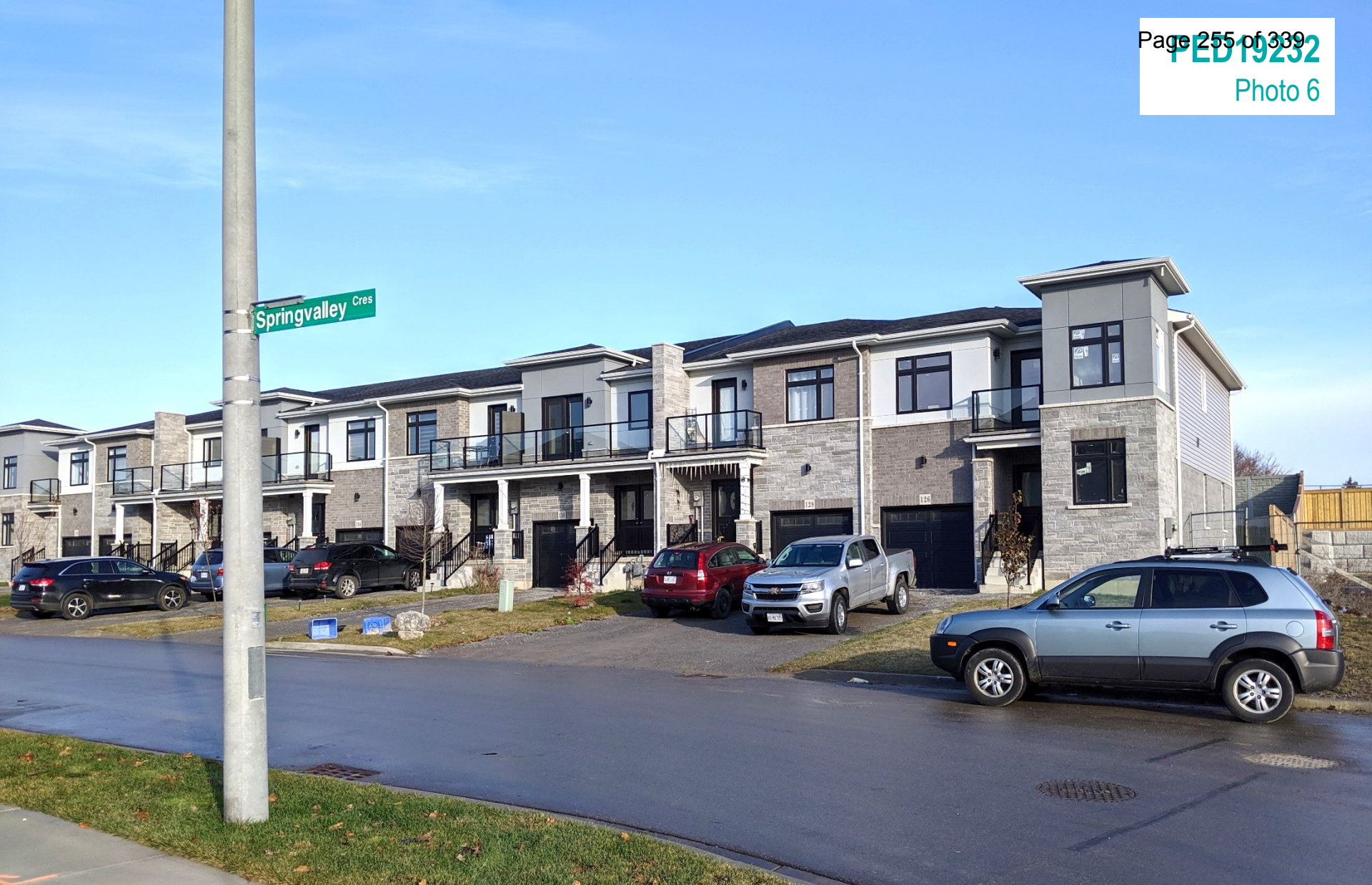
Street townhouses along Springvalley Crescent, northwest of Subject Lands
