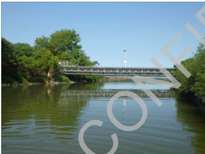
Facing downstream from east bank.
