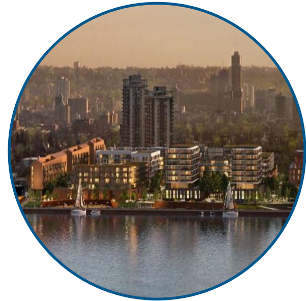
1,700 m of New Utilities
