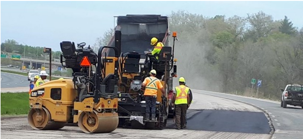
205 Lane km Resurfacing
