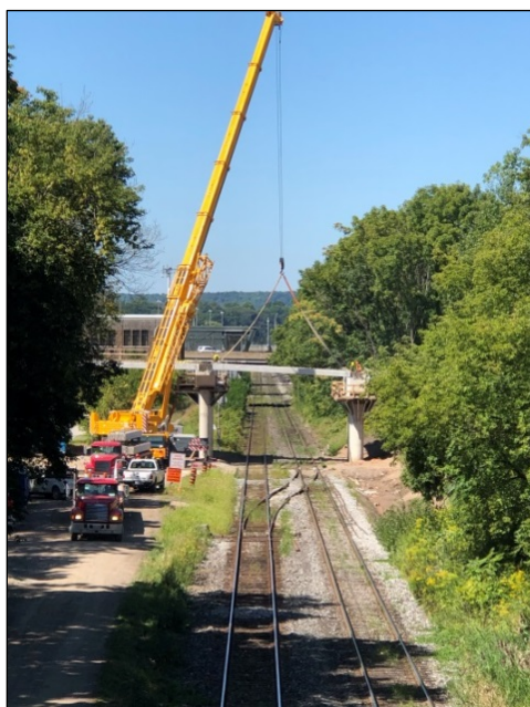
Widening the John Street bridge allows us to expand GO Train service to Hamilton
