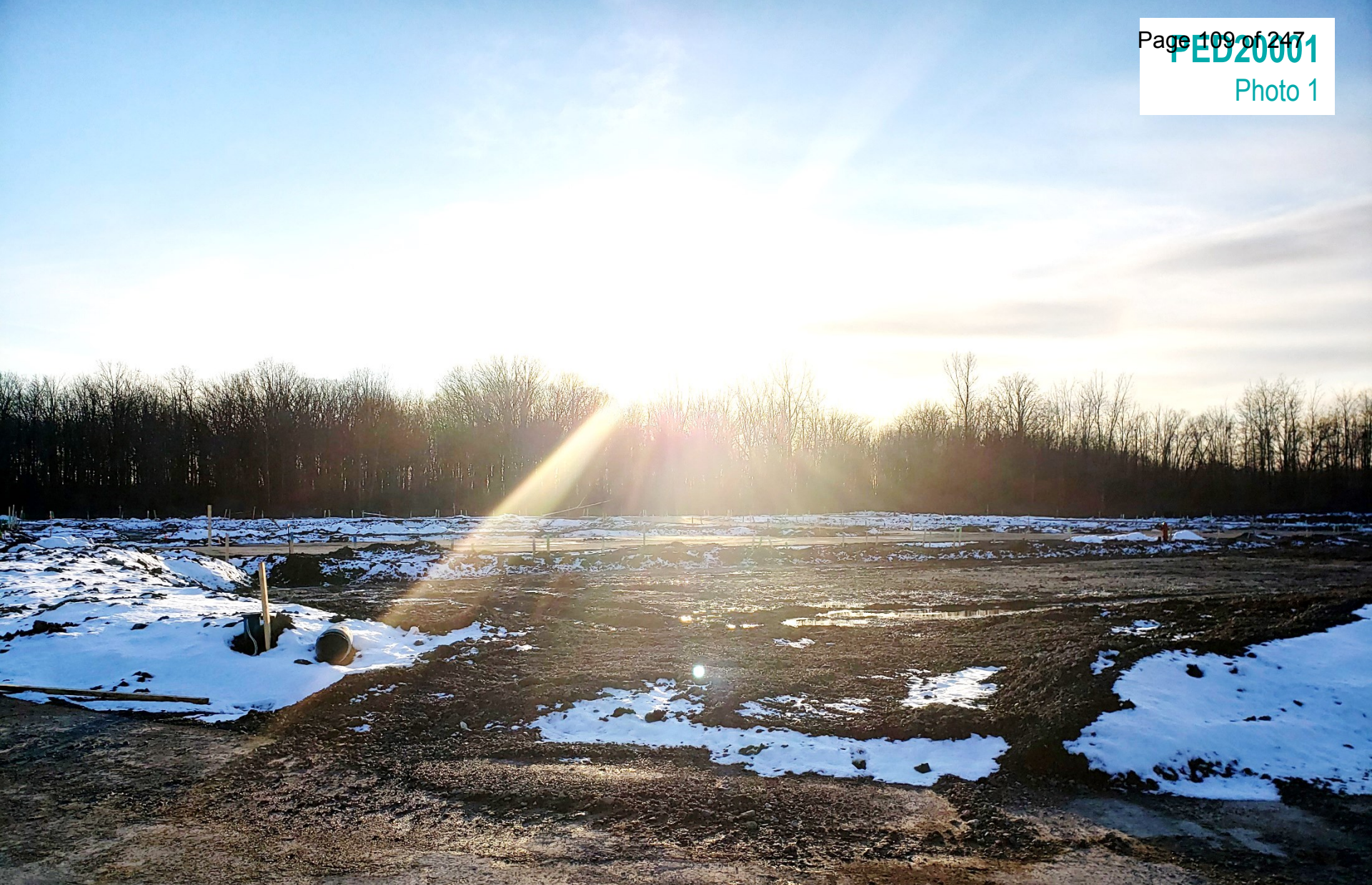
Subject Lands, wood lot to the south
