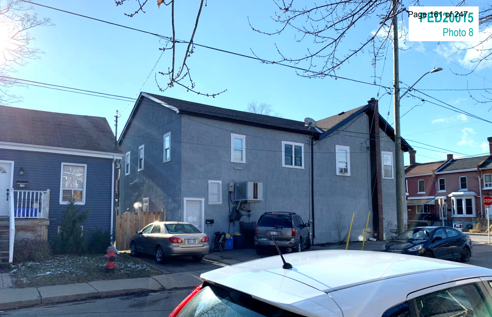
South side of Robert Street, looking west
