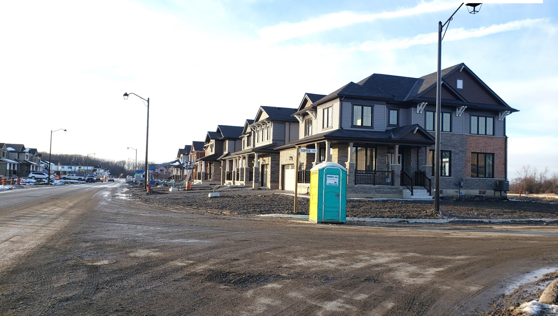
Existing Townhouses to the north
