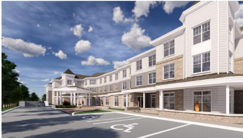
MAIN ENTRANCE LOOKING NORTH
