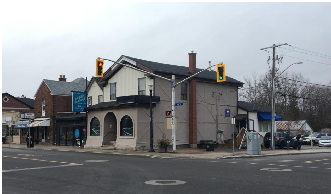
Image 2: View towards northeast corner of King Street East and Mountain Avenue North showing the south façade of 23 & 25 King Street East and the east façade of 25 King Street East, Stoney Creek (MB, 2020).
