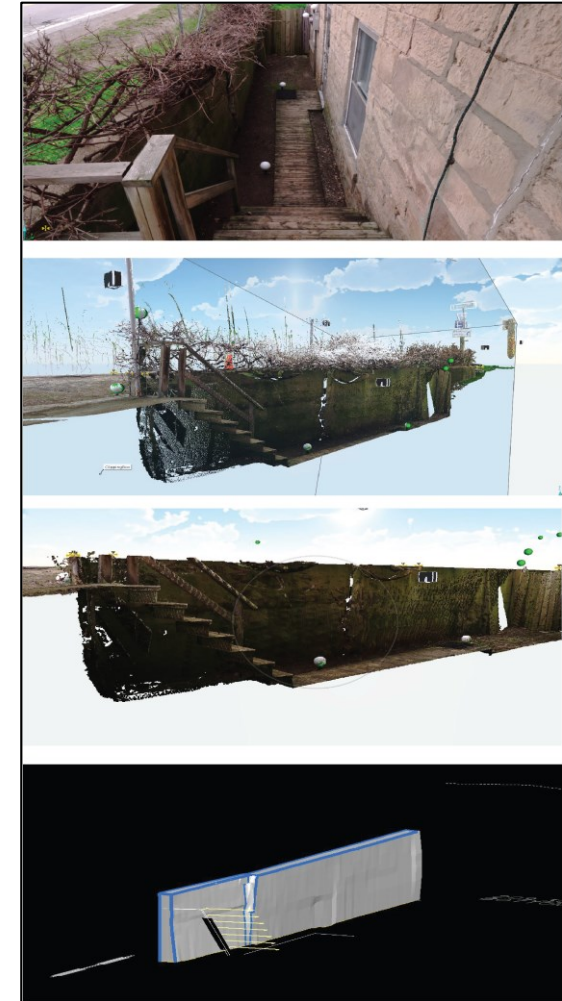
LIDAR Technology (Hwy 8 & Brock Rd)
