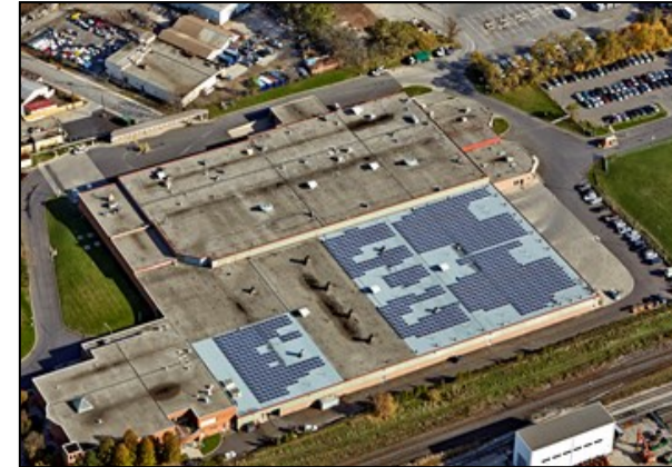
Solar panels-Wentworth Operations Centre
