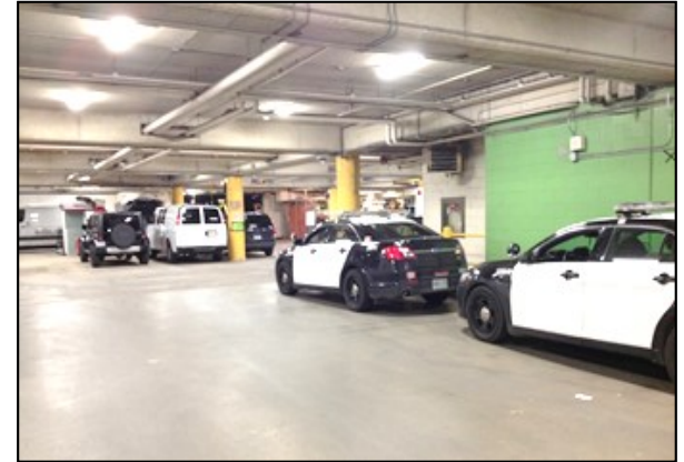
LED Lighting Retrofit
