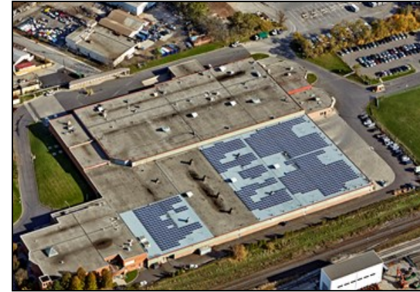
Solar panels-Wentworth Operations Centre
