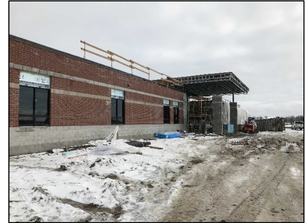
Beverley Community Centre - Construction
