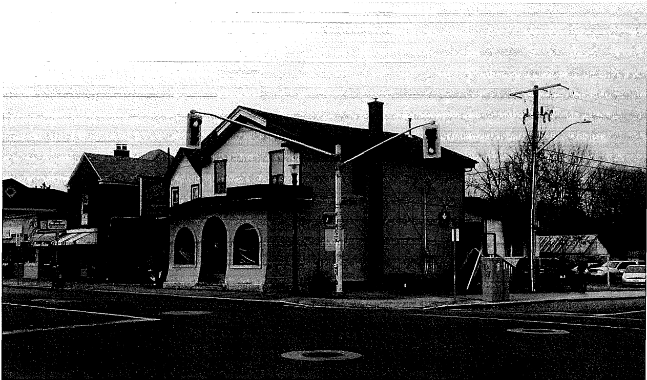
Image 2: View towards northeast corner of King Street East and Mountain Avenue North showing the south façade of 23 & 25 King Street East and the east façade of 25 King Street East, Stoney Creek (MB, 2020).
