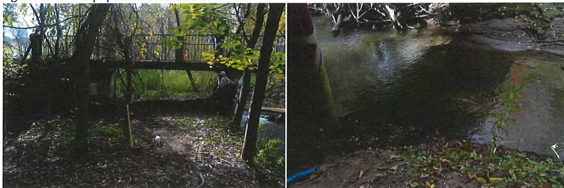
Figure 4: AC-1 equipment installation
