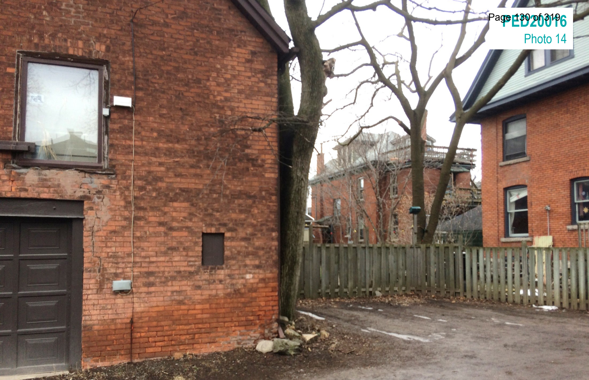
Parking area and existing accessory building locate to the north of the subject property, as seen from the alleyway looking north
