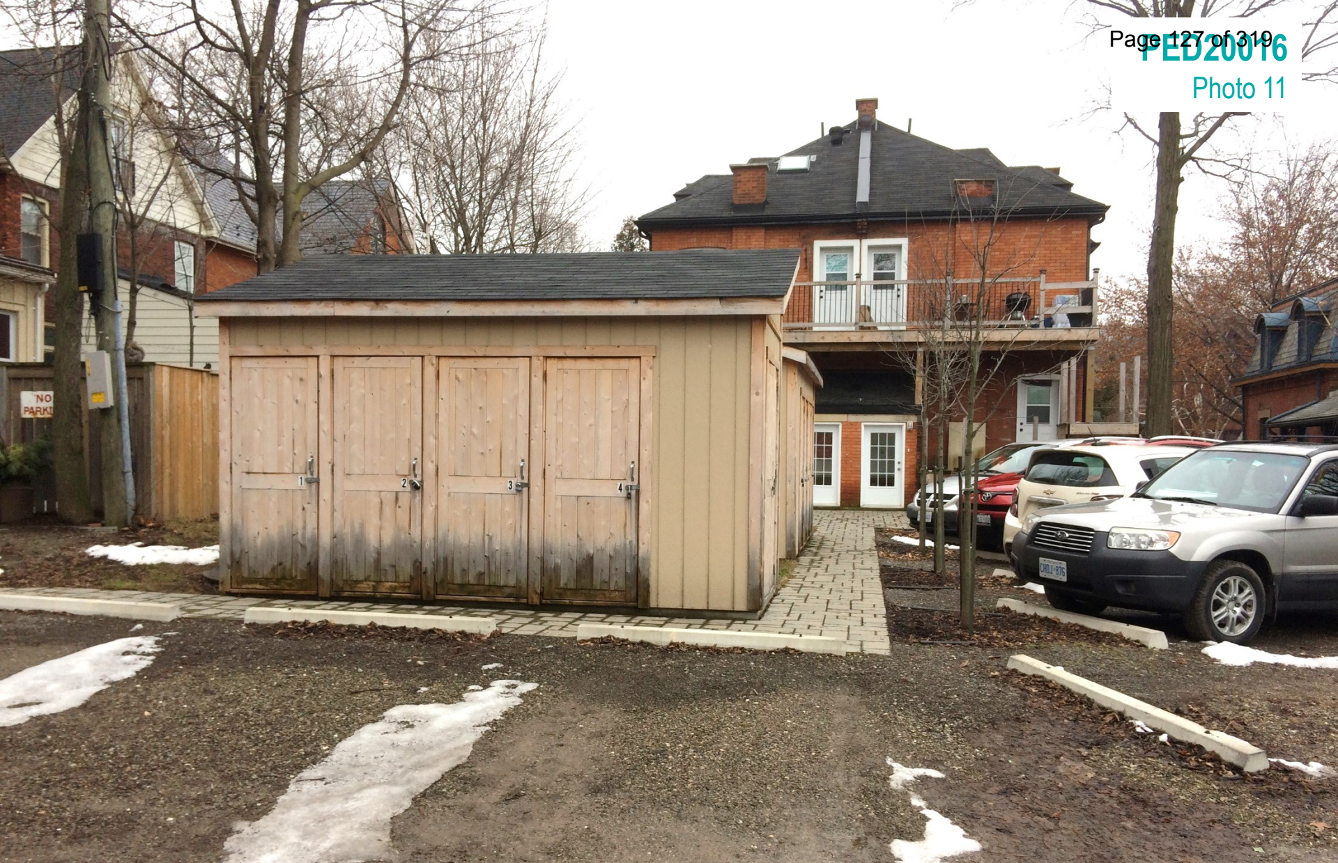
Parking spaces and accessory building located at the rear of the subject property, as seen from the alleyway looking south
