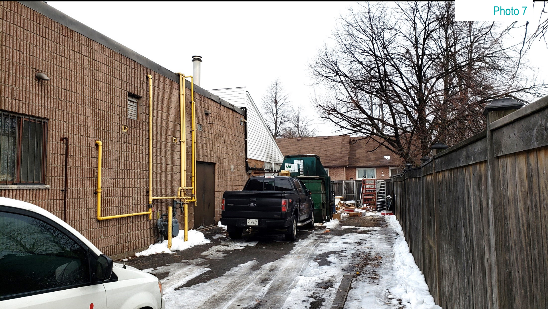
Freezer addition from south
