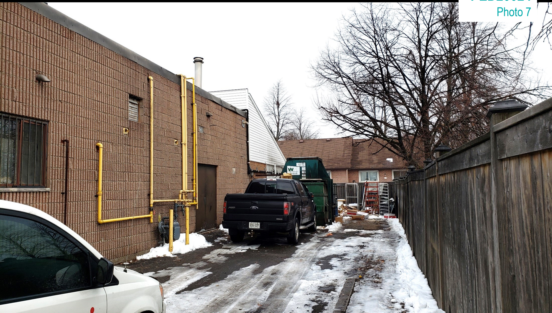
Freezer addition from south
