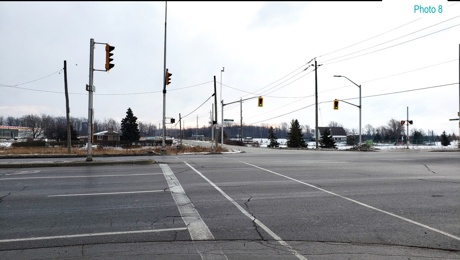
View to the east along Green Mountain Road
