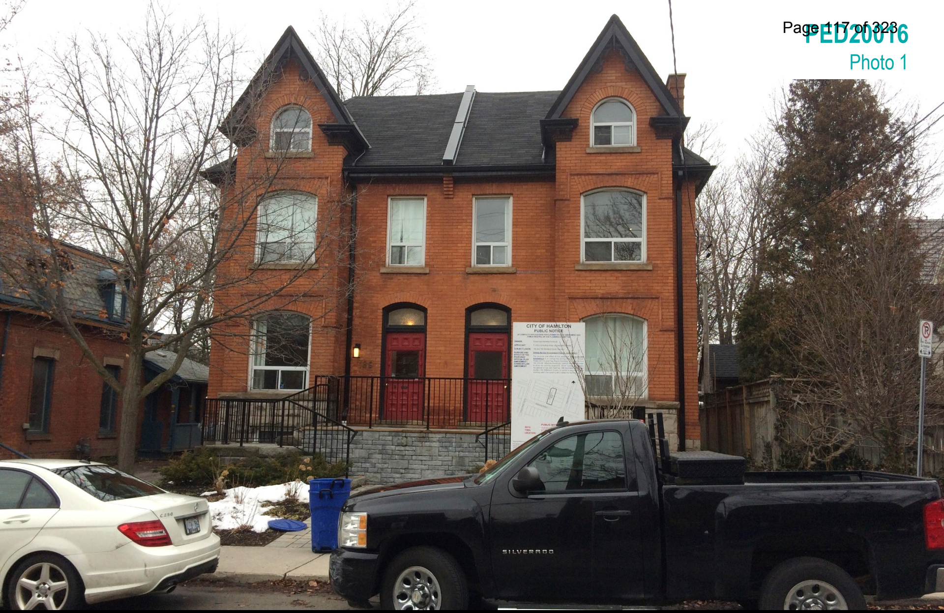
Subject property, as seen from Markland Street looking north
