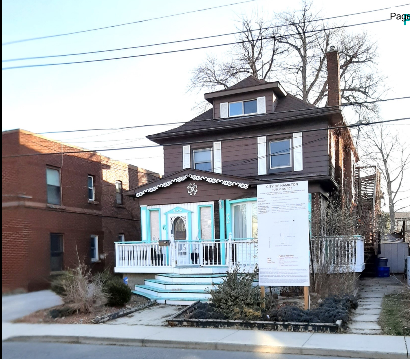
Subject property looking east on Grosvenor Avenue South
