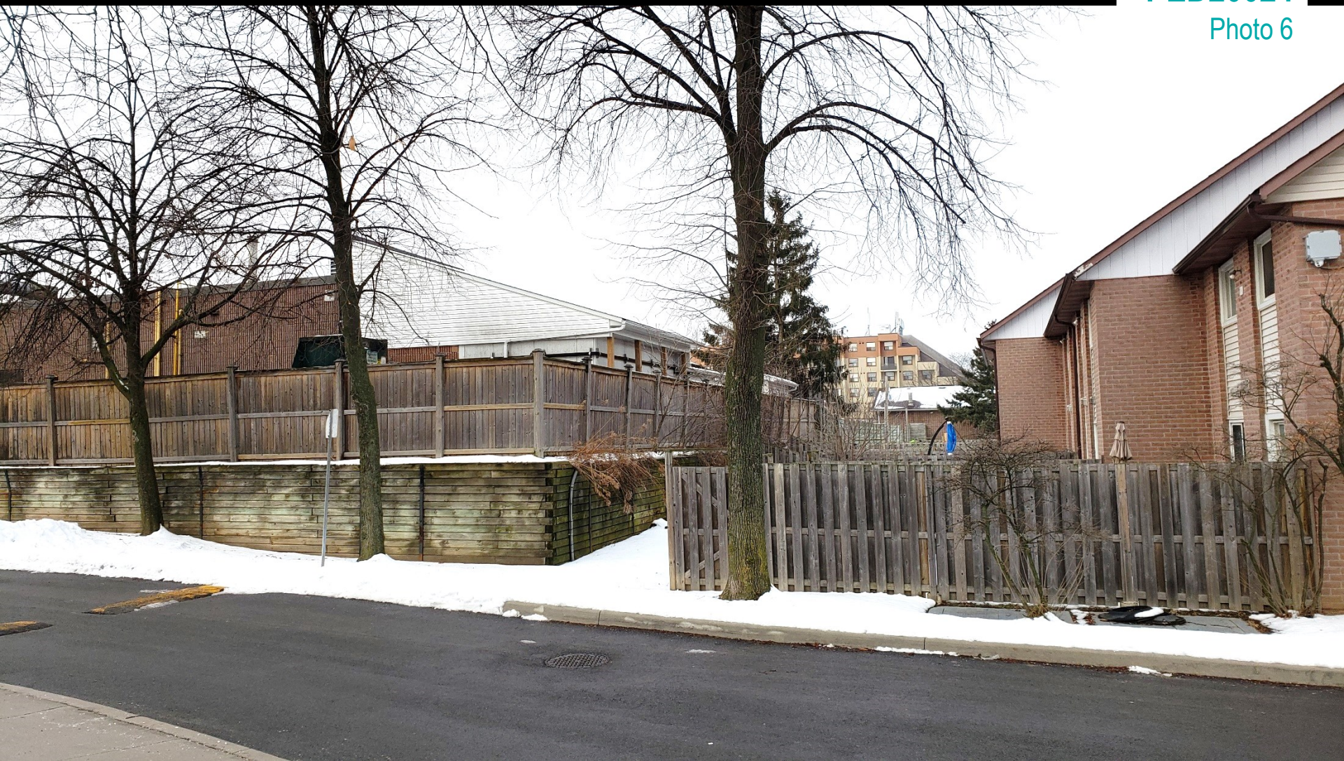
Freezer addition from east
