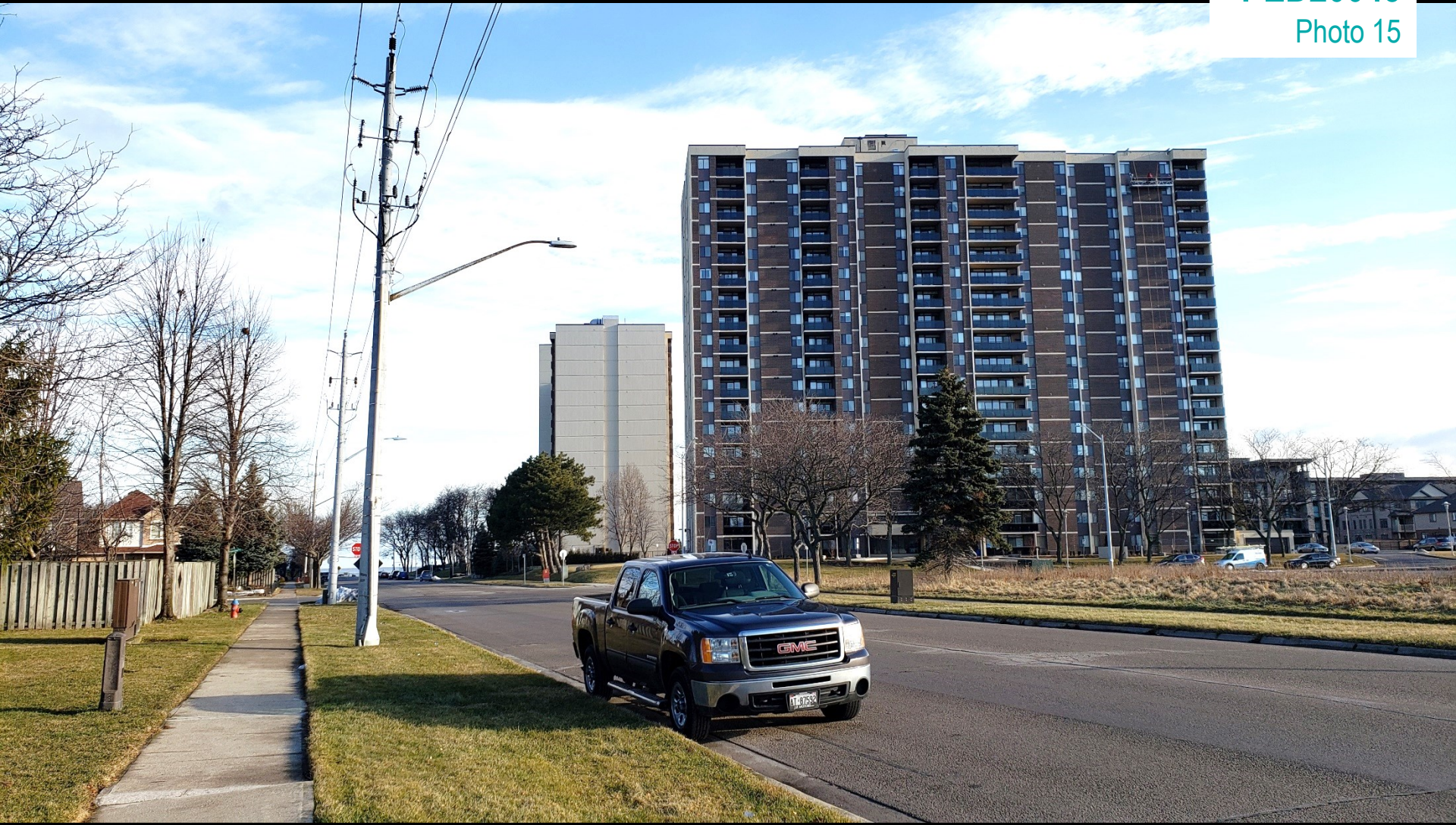
Existing multiple dwellings north of Frances Avenue
