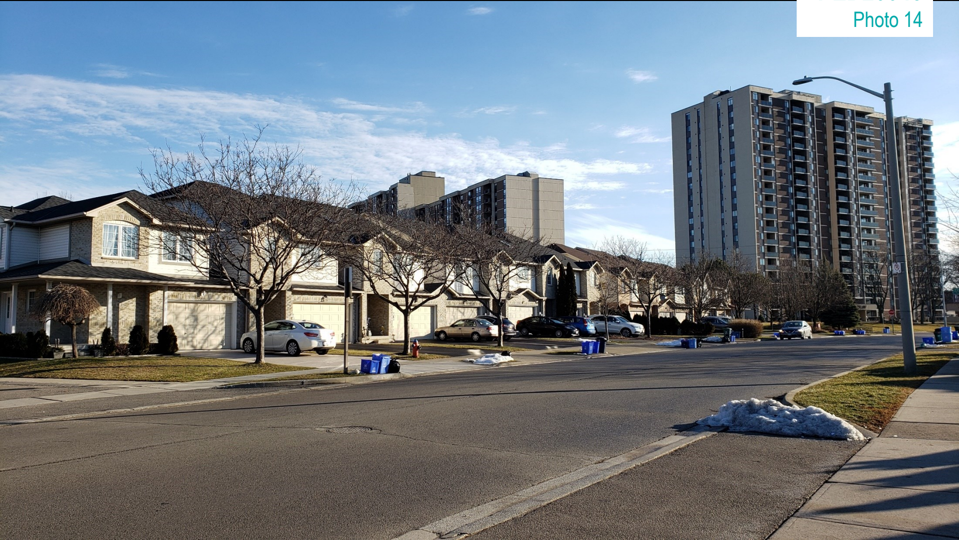
Existing street townhouses and multiple dwellings north of Frances Avenue
