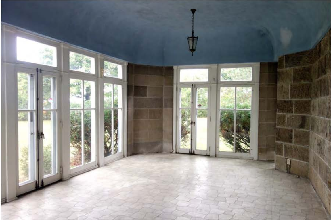
SUNROOM – unheated with no basement, solid masonry walls with no insulation, glazing on three sides
