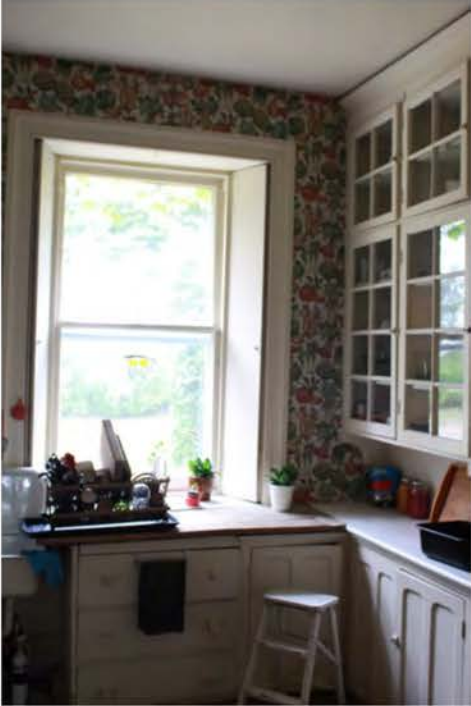
PANTRY – built-in cabinets
