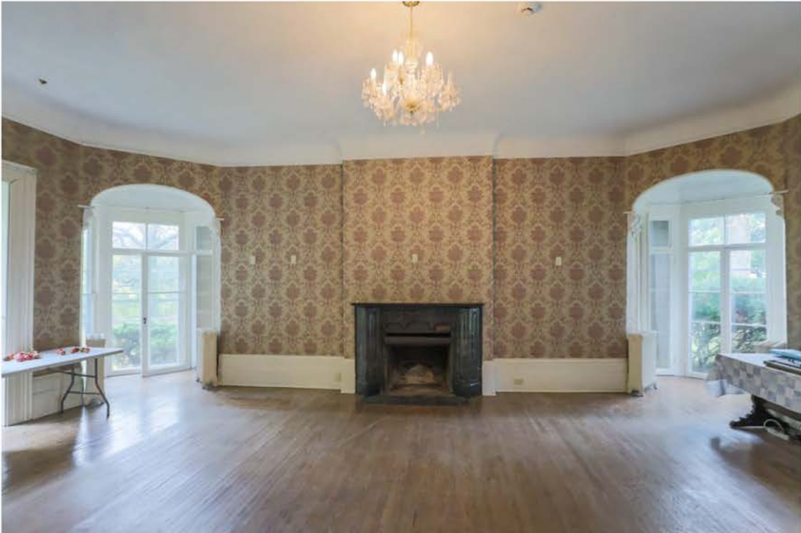
BALLROOM – wood floors, wood trim, wood windows, plaster & lathe, wallpaper, marble fireplace
