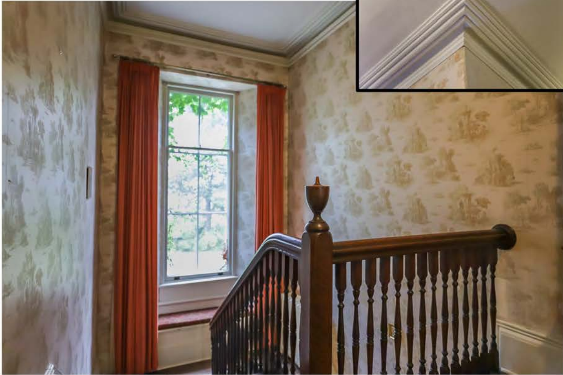
MAIN STAIRCASE – stained oak banister, wood trim, plaster crown moulding, wallpaper
