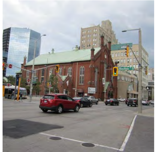
Brick Pinnacles & Buttresses
