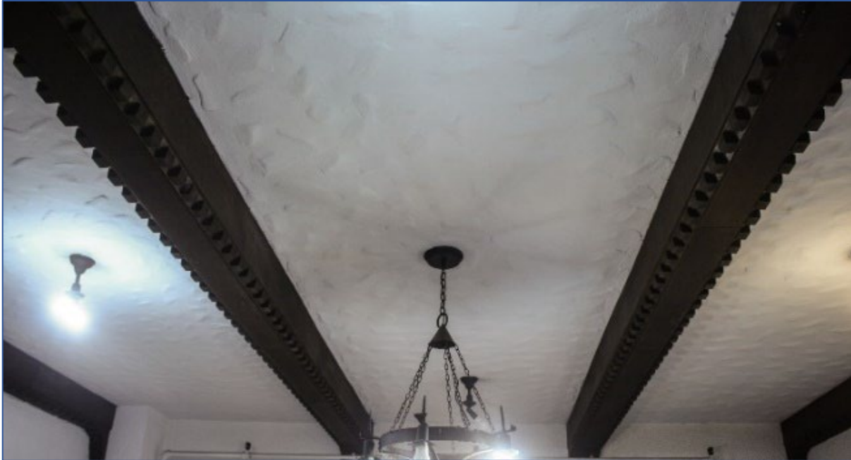
Figure 42: Ceiling of the foyer (AB, 2018).
