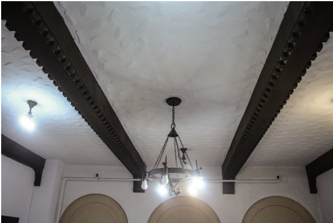
Figure 33 Foyer – wood rafters across ceiling, metal chandelier (ZH, 2018).
