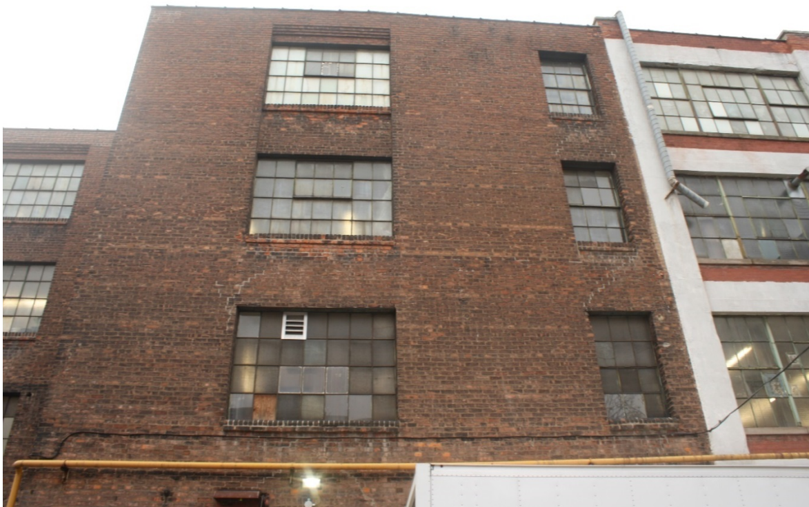
Figure 10 South side wall transition between east (right) and west (left) sections (ZH, 2018).
