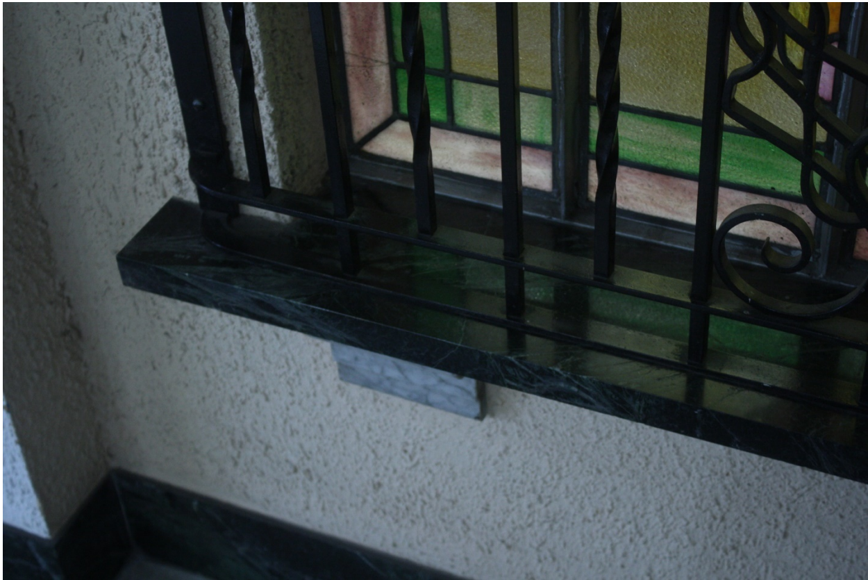
Figure 40 Foyer – showing indoor window sill in black marble supported by white marble brackets (ZH, 2018).
