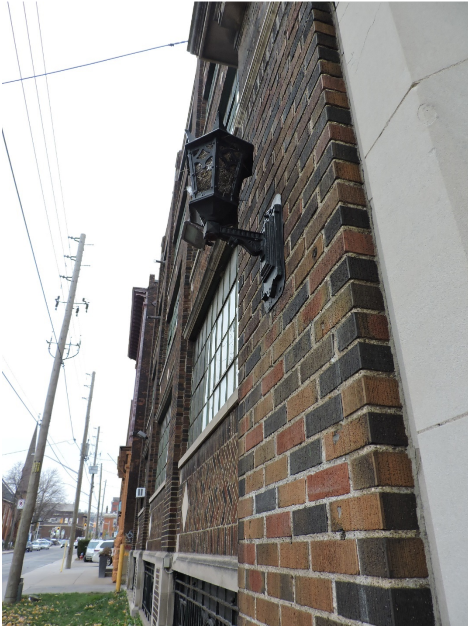
Figure 18 Front façade showing metal lamp detail; streetscape looking south (AB, 2018).
