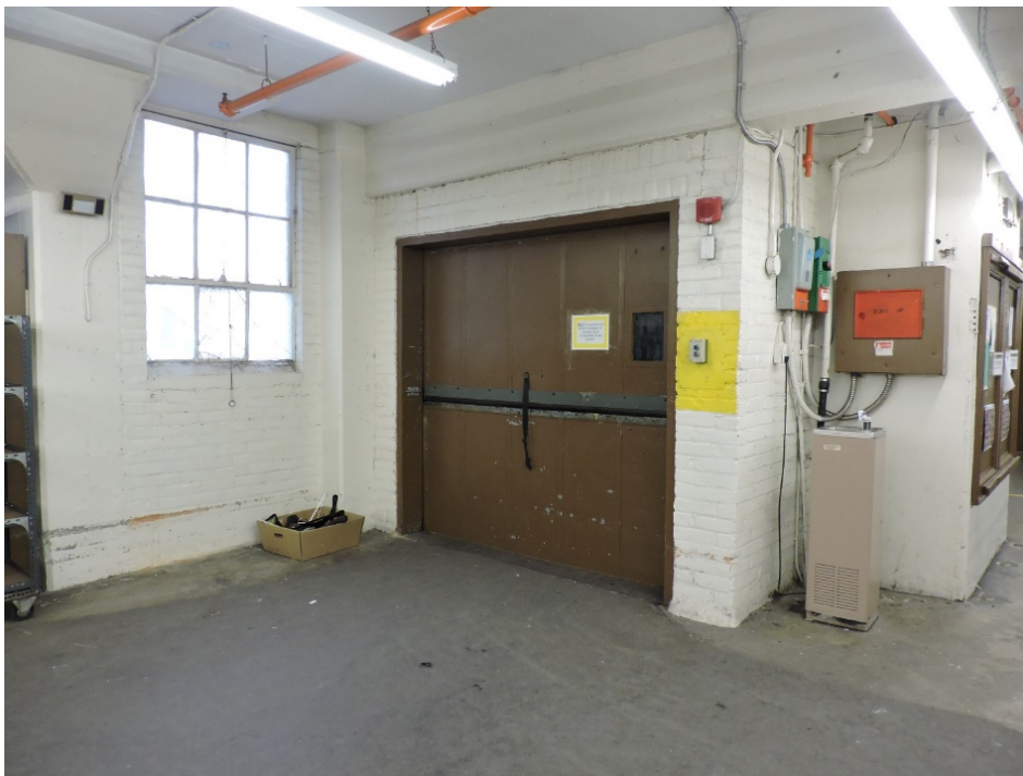
Figure 56: Fourth floor, elevator (AB, 2018).
