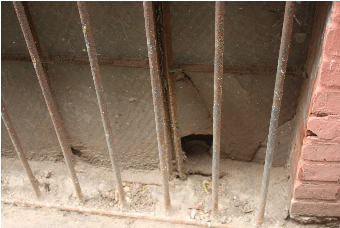
Figure 9 Deteriorating barred basement windows on south wall of the east section (ZH, 2018).
