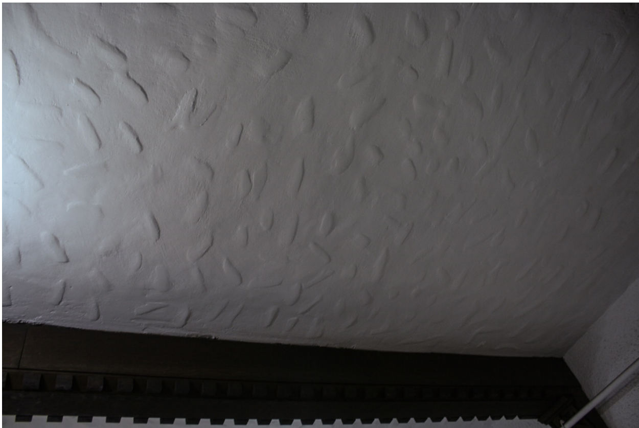
Figure 39 Foyer – showing patterned plastered ceiling (ZH, 2018).
