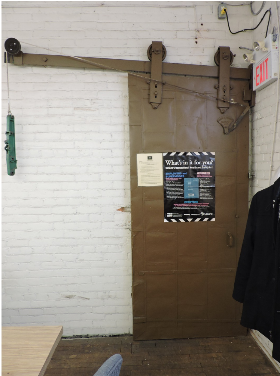
Figure 56 Fire door leading to staircase in west section (AB, 2018).
