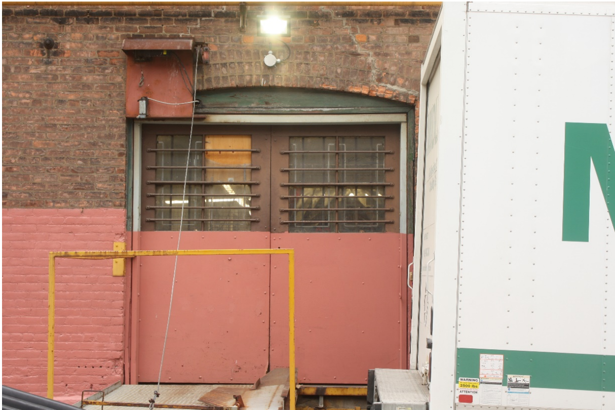
Figure 11 Bay door on south side of west section (ZH, 2018).
