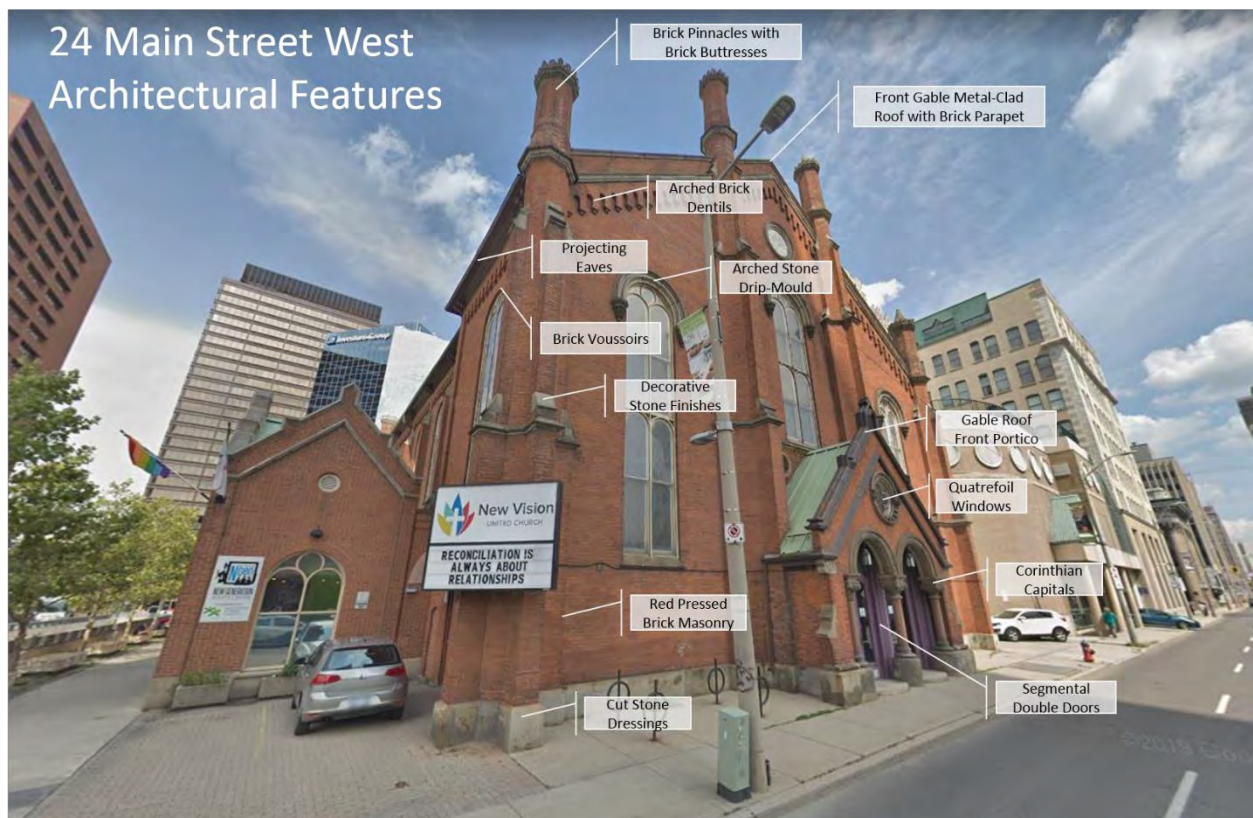
Image 8 – Visual of Significant Exterior Architectural Features. (Source: Google Maps).
