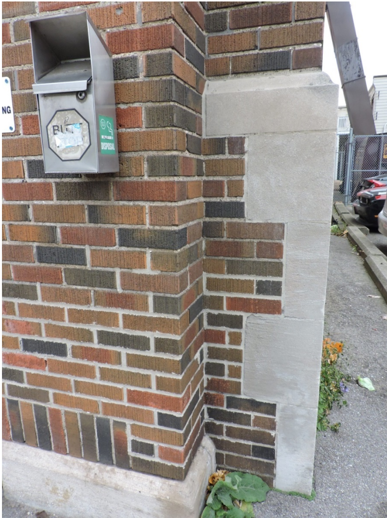
Figure 21 Northeast corner of east section showing concrete/stone quoins (AB, 2018).
