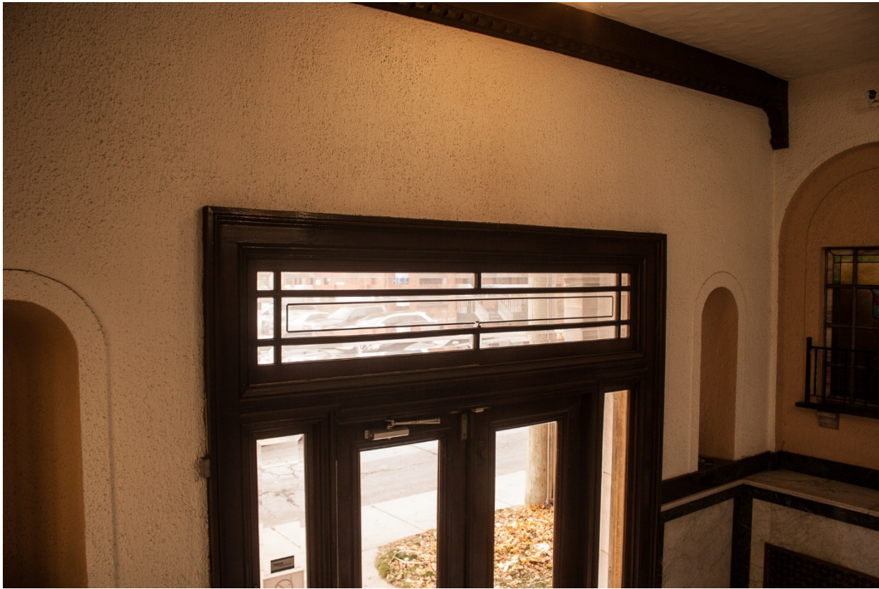
Figure 38 Foyer – showing both niches and detail of transom light above doorway (ZH, 2018).
