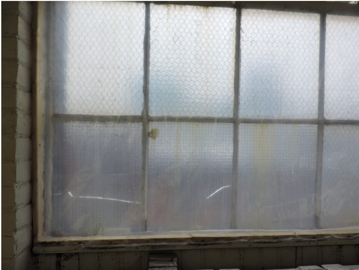
Figure 57 Interior window detail (AB, 2018).
