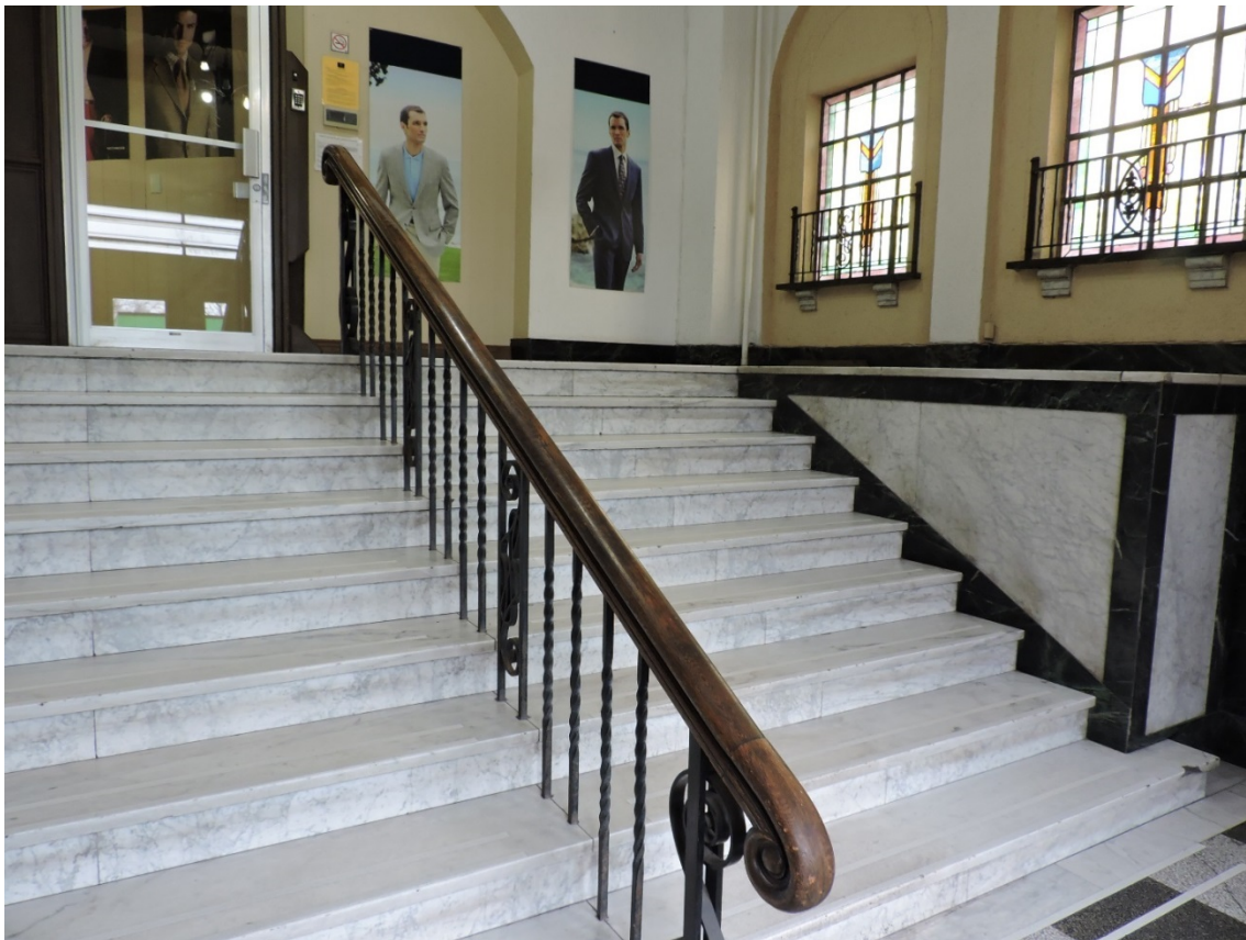
Figure 31 Foyer – marble staircase with wood and metal railing (ZH, 2018).
