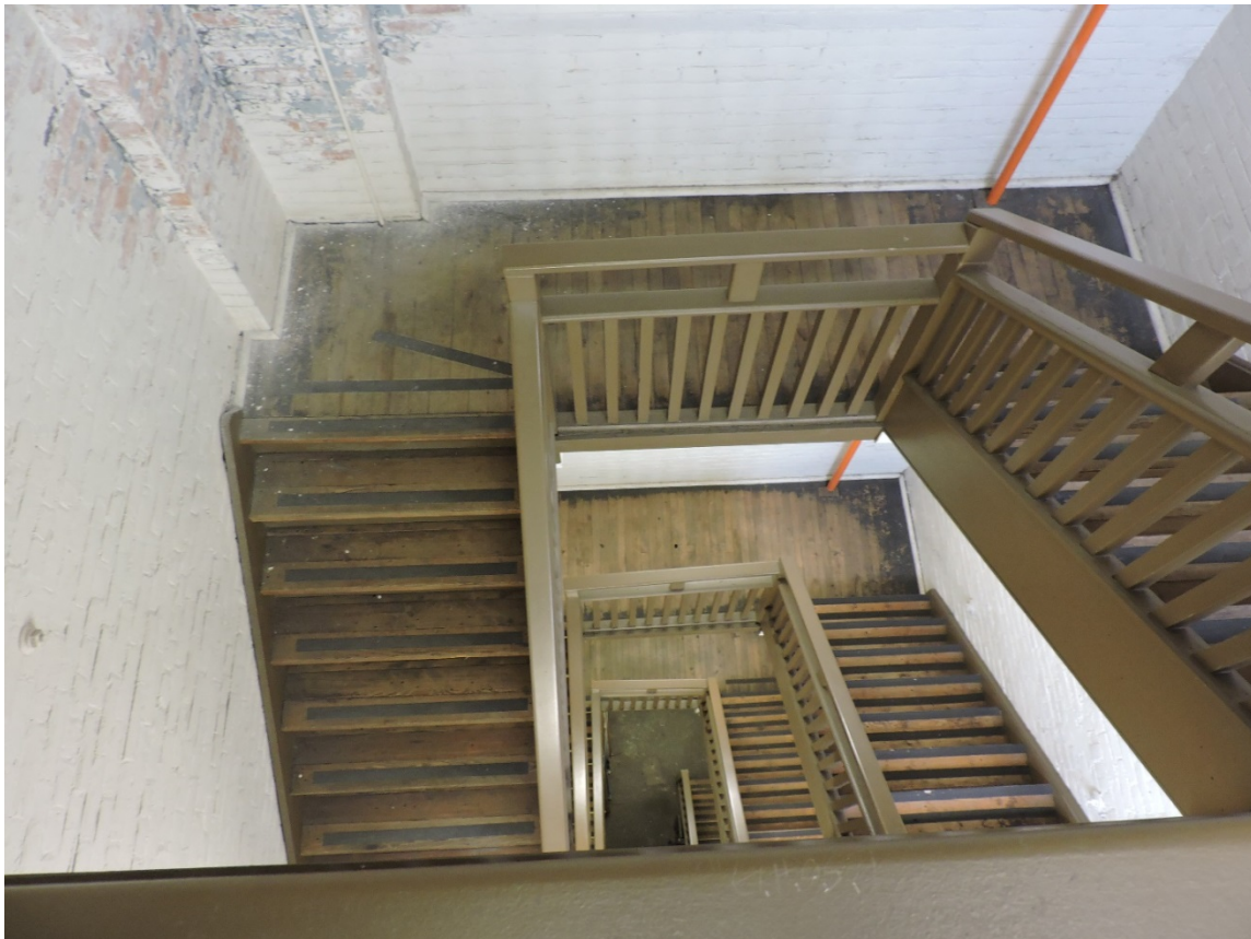
Figure 58 West section staircase (AB, 2018).
