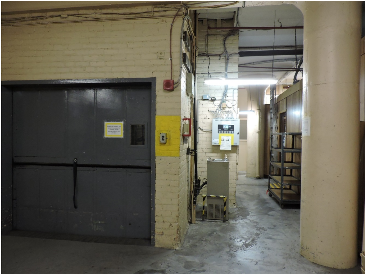
Figure 72 Bay door in east section (AB, 2018).
