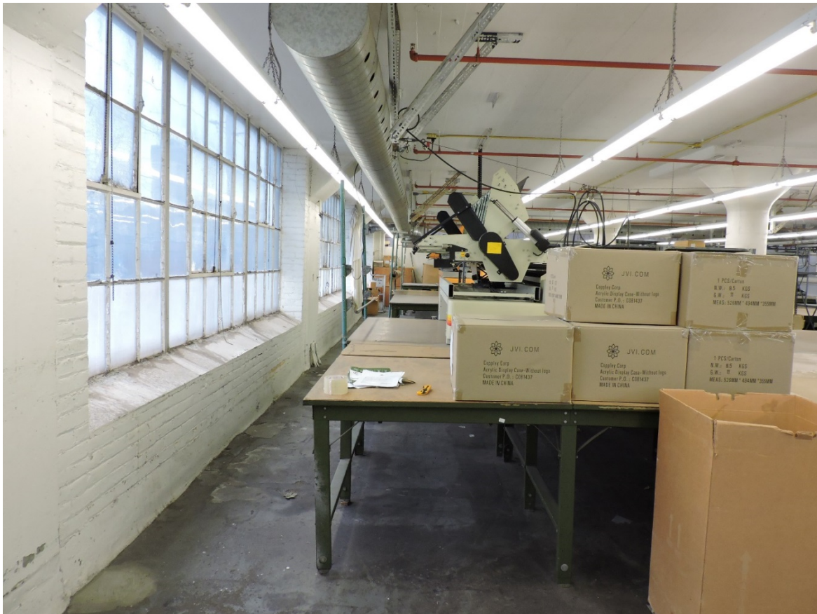
Figure 62 East section interior showing inner window details and concrete floor (AB, 2018).
