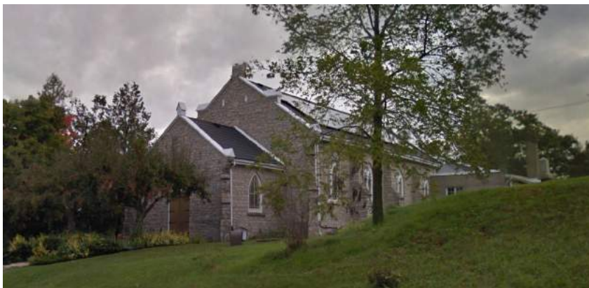
Figure 5.14- West Flamborough Presbyterian Church (source - google maps)
