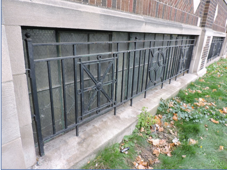
Figure 35: Metalwork located along basement level (AB, 2018).
