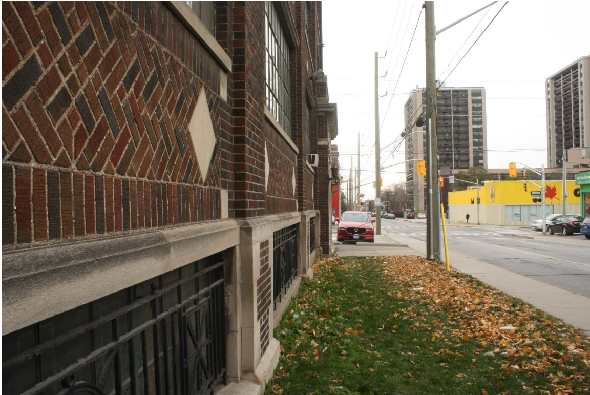
Figure 15 Front façade showing streetscape looking north on Hughson Street North, brick weave bond details, and barred front basement windows (ZH, 2018).
