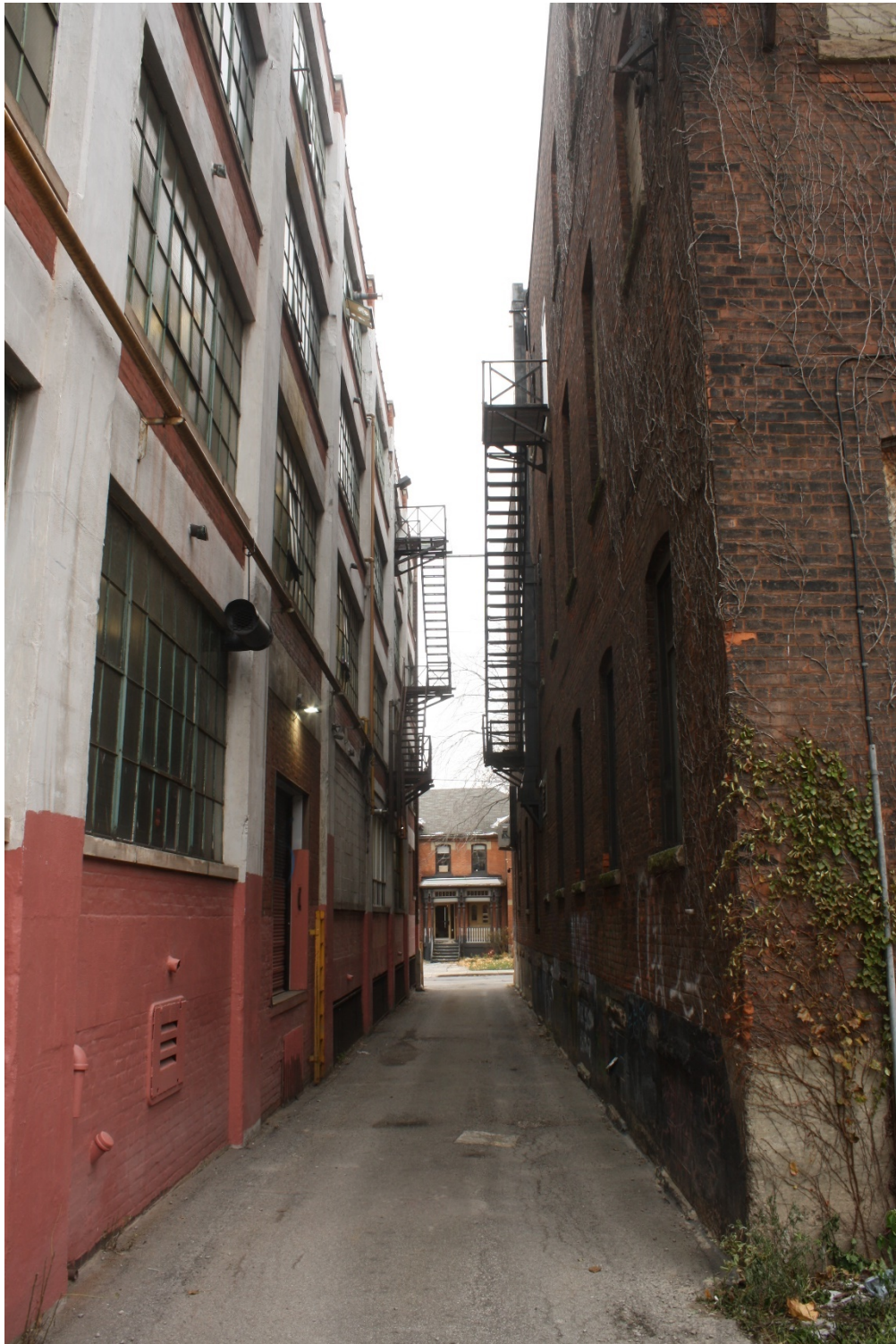
Figure 8 Alleyway on south side of subject property, looking east (ZH, 2018).
