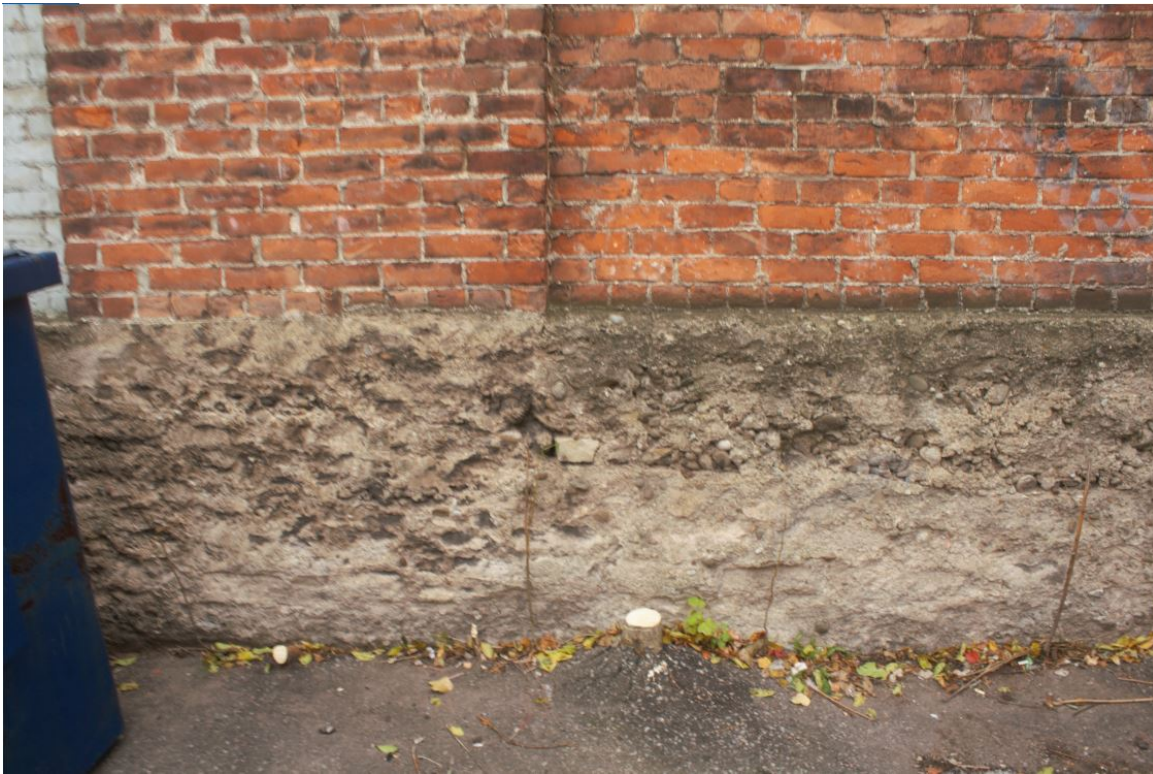
Figure 26 West section concrete foundation on north façade (ZH, 2018).
