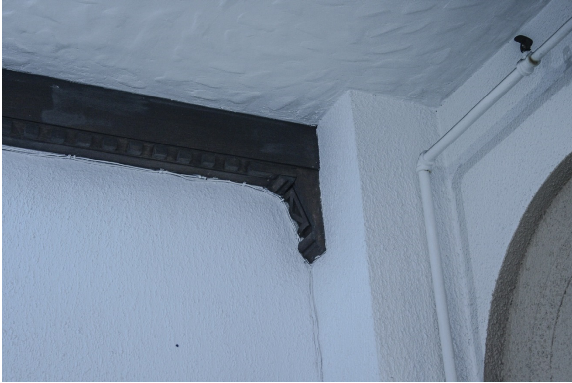
Figure 32 Foyer – wood rafter with carved dentils and decorated brackets (ZH, 2018).
