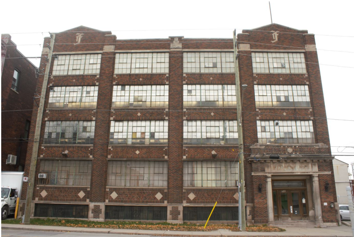
Figure 6 Front façade of subject property (ZH, 2018).
