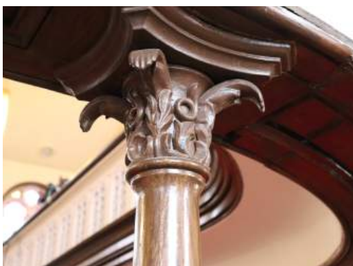
Figure 4.14 - Detail of Column supporting balcony
