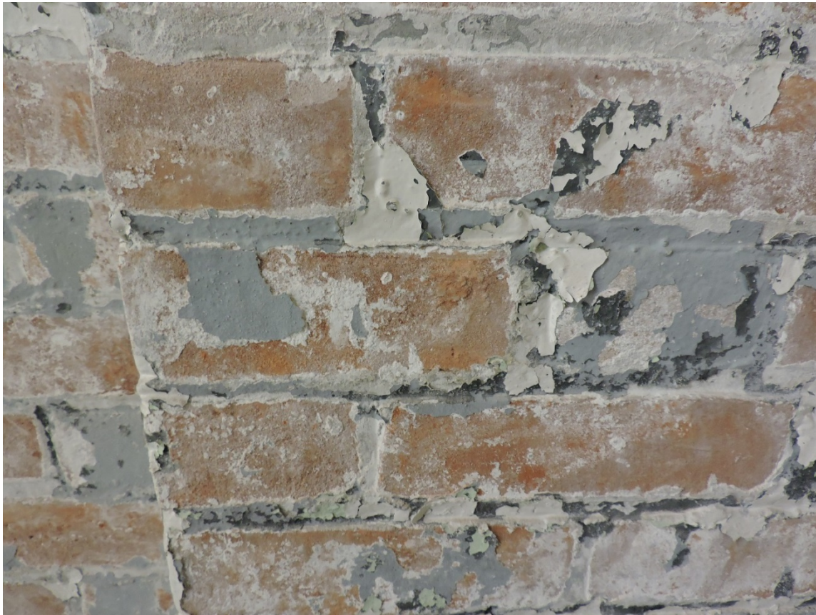
Figure 59 Brick condition in staircase (AB, 2018).
