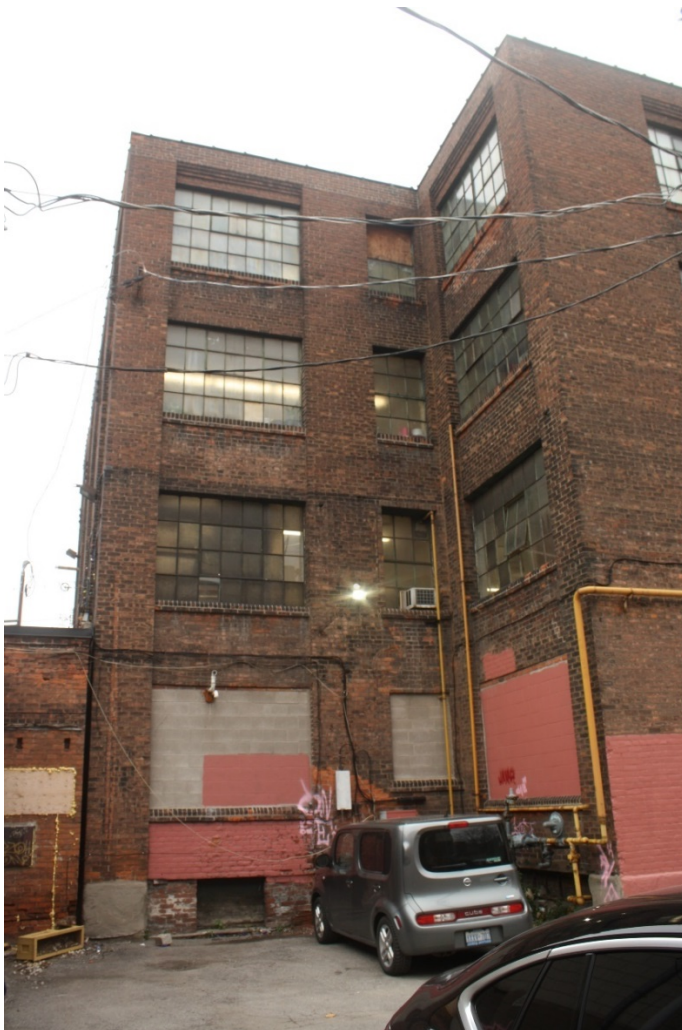
Figure 14 Southwest corner of the west section showing sealed bay doors and one-story connection to shops (ZH, 2018).
