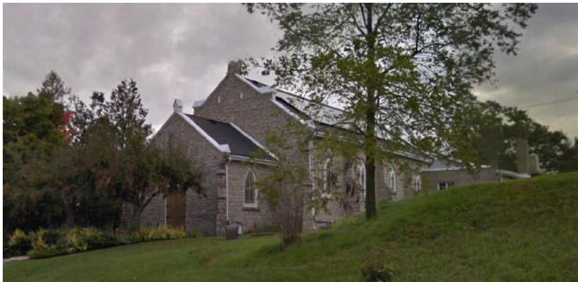
Figure 5.14- West Flamborough Presbyterian Church (source - google maps)
