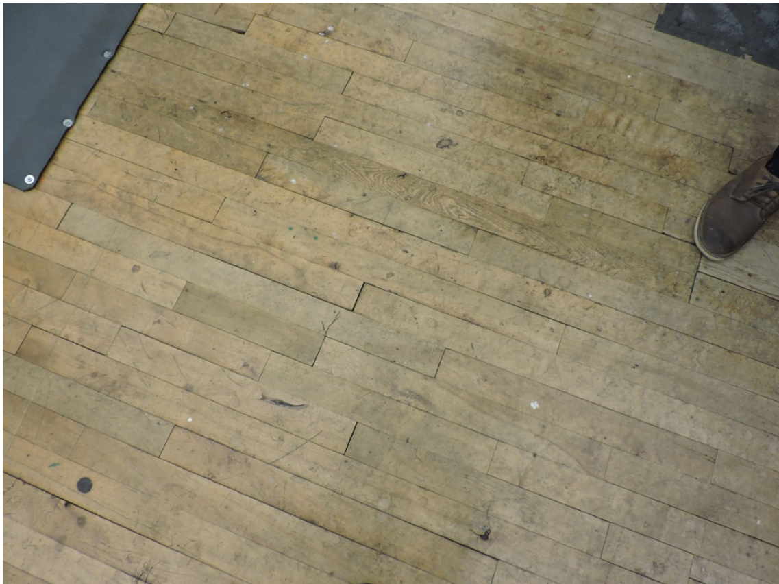
Figure 53 Detail of wood plank floors, west section (AB, 2018).
