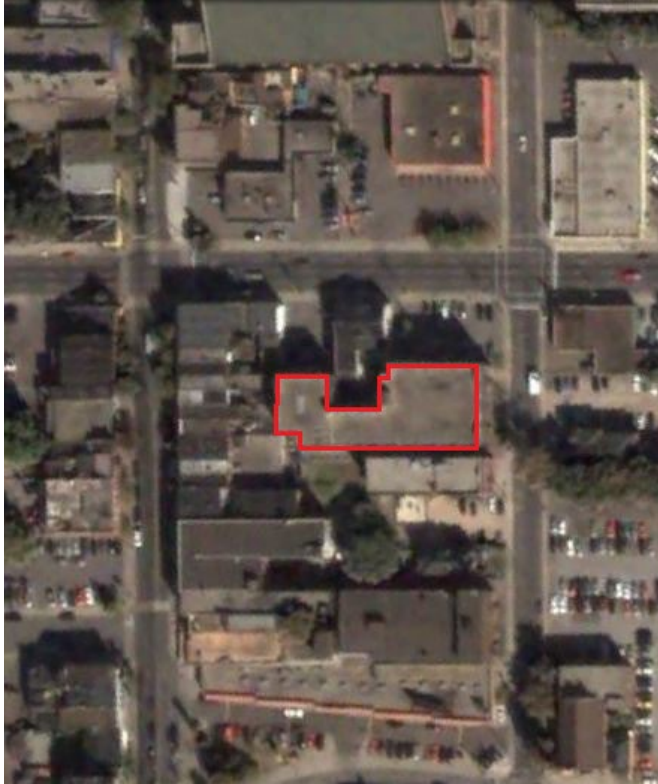
Figure 27: Satellite photograph of the subject building and vicinity. Subject property's structure outlined in red (Google Earth, 2004).
