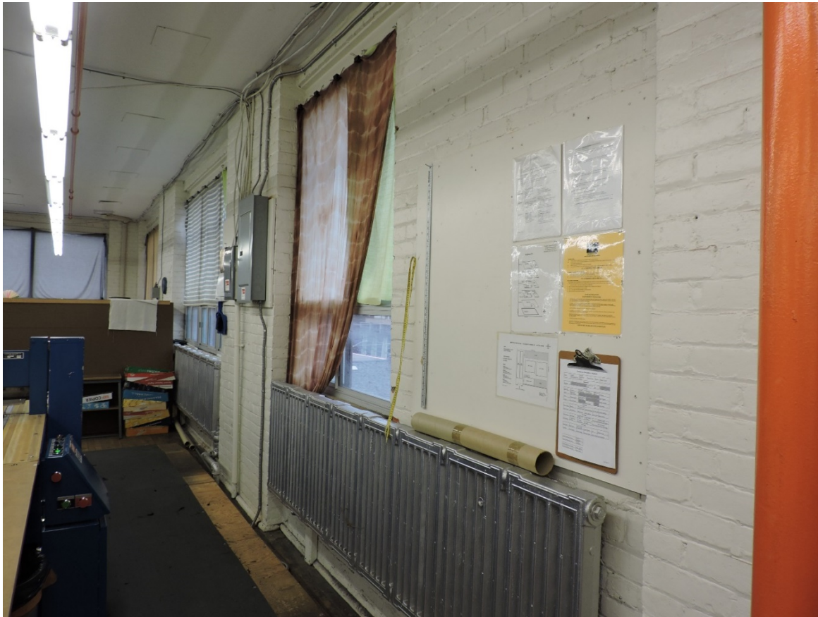
Figure 54 West section – painted white brick across interior of building (AB, 2018).
