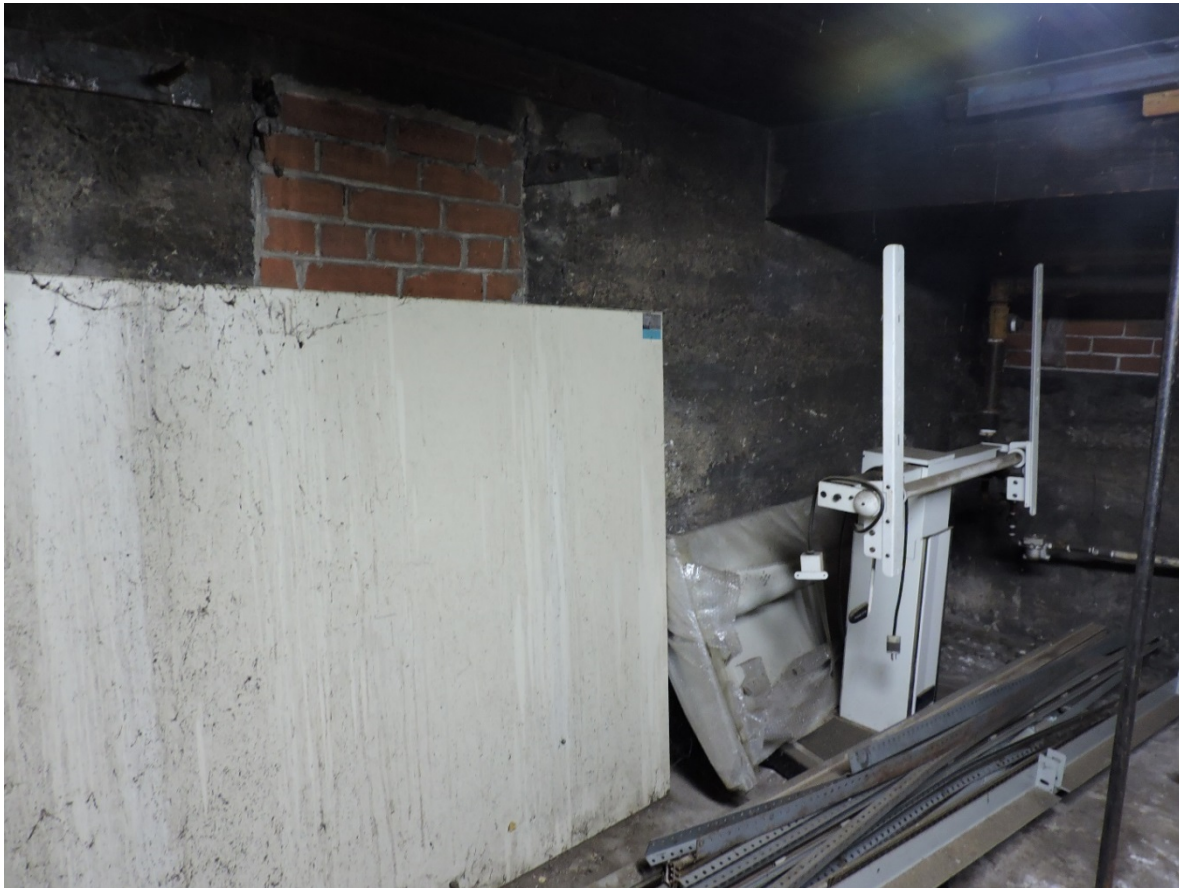
Figure 65 Basement of west section showing concrete foundation and sealed windows (AB, 2018).
