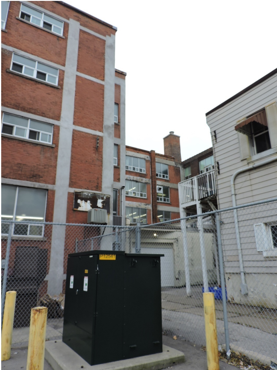
Figure 23 North stepped façade of east section transitioning to west section (AB, 2018).
