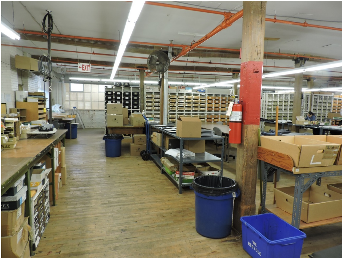
Figure 52 West section showing wood plank floors and wood pillars (AB, 2018).
