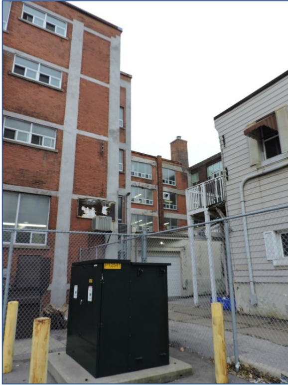
Figure 37: North elevation where two buildings meet (AB, 2018).
