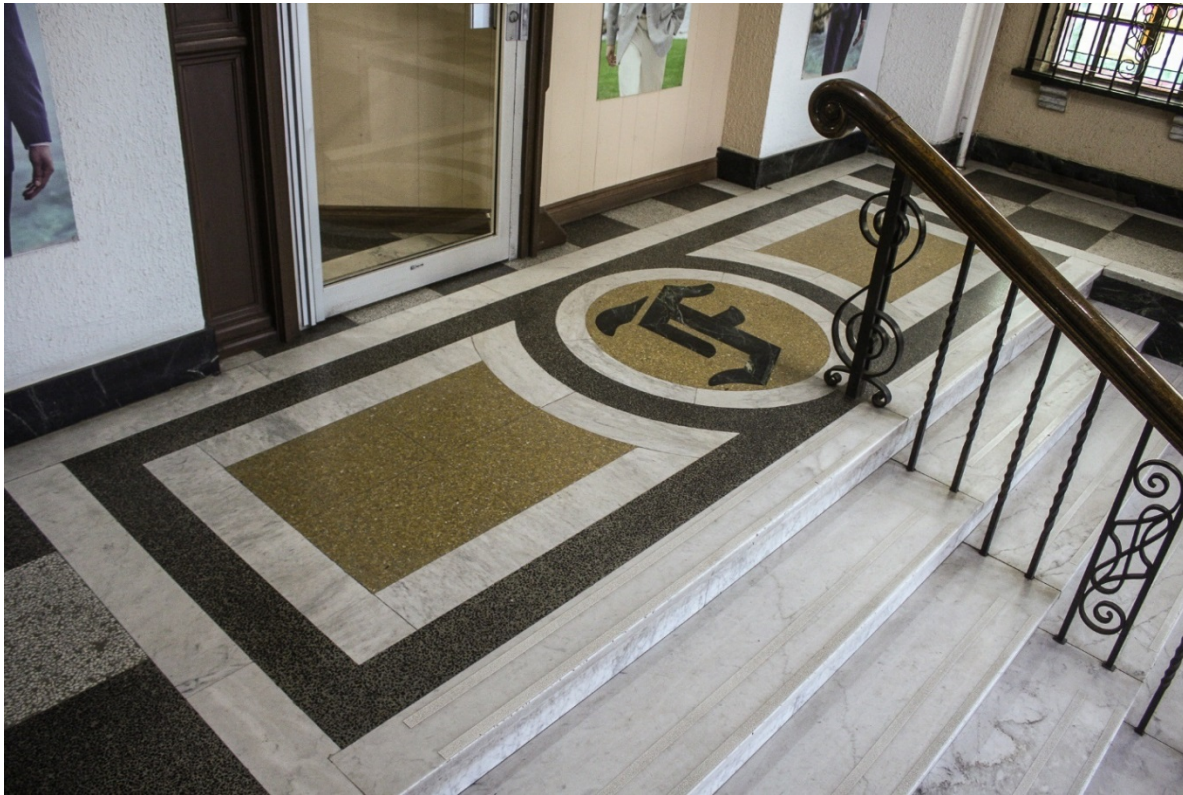
Figure 34 Foyer – decorative pebbled tile mixed with marble trim in an ‘F’ design before the first level’s front door (ZH, 2018).
