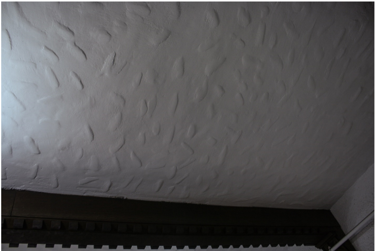
Figure 39 Foyer – showing patterned plastered ceiling (ZH, 2018).
