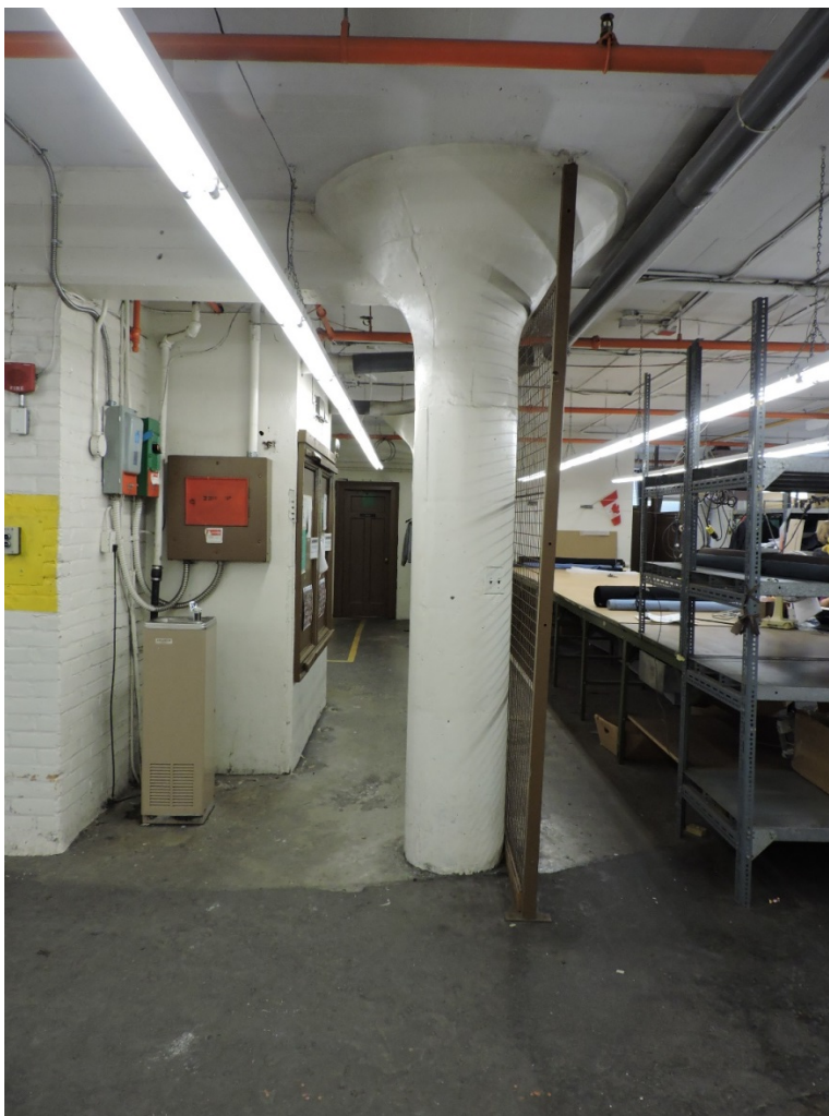
Figure 47 Metal pillar of east section (AB, 2018).
