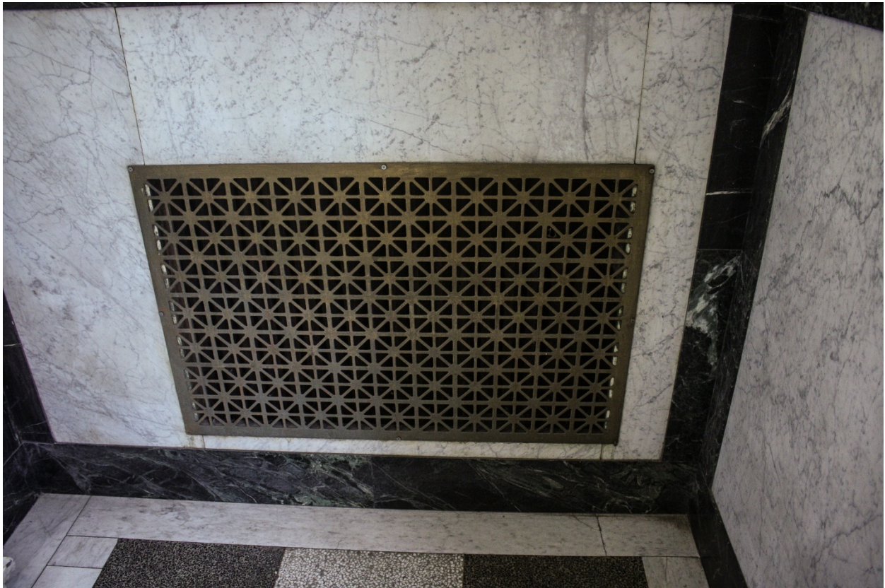
Figure 41 Foyer – showing metal grate on the lower split level (ZH, 2018).
