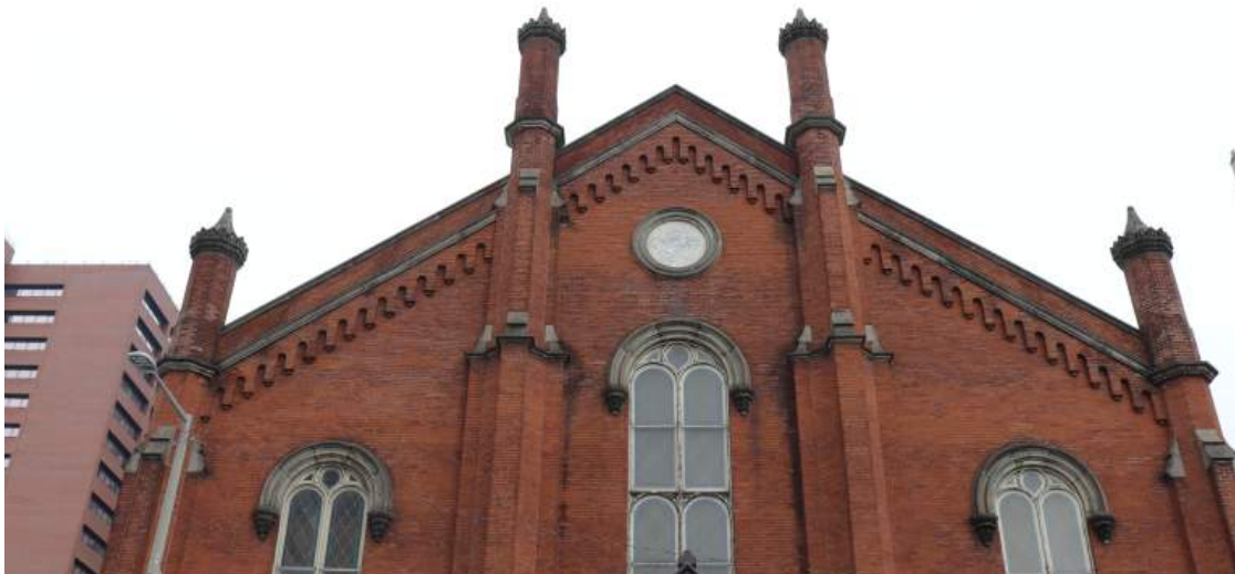
Figure 4.9 South Elevation - top showing castellations
