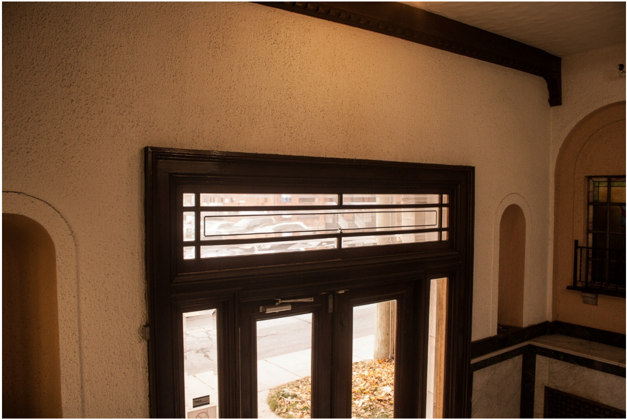
Figure 38 Foyer – showing both niches and detail of transom light above doorway (ZH, 2018).
