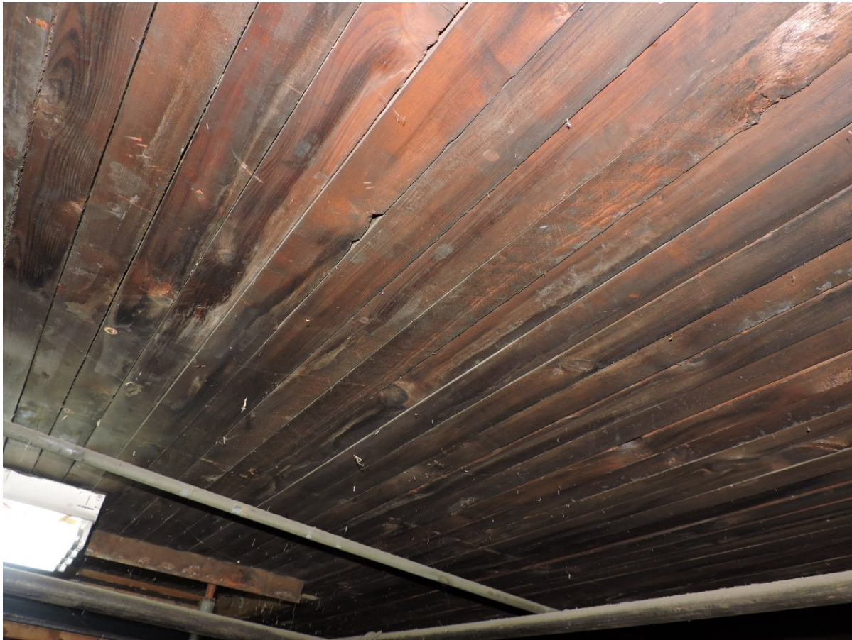
Figure 67 Basement level of west section showing wood plank ceiling (AB, 2018).
