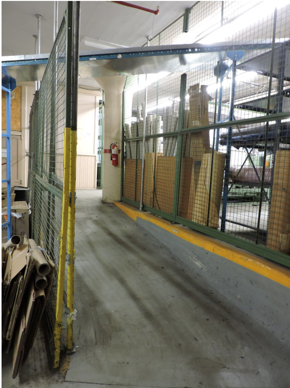
Figure 71 Ramp on main level (AB, 2018).
