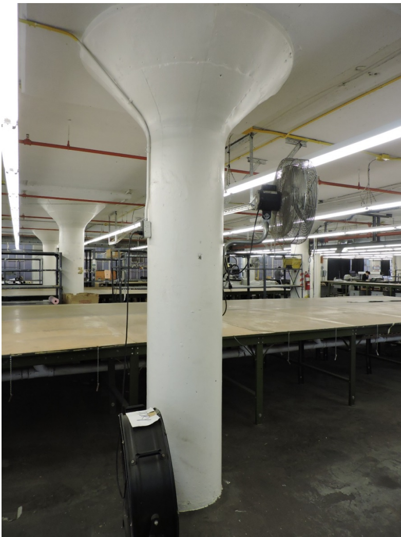
Figure 64 East section metal pillar (AB, 2018).
