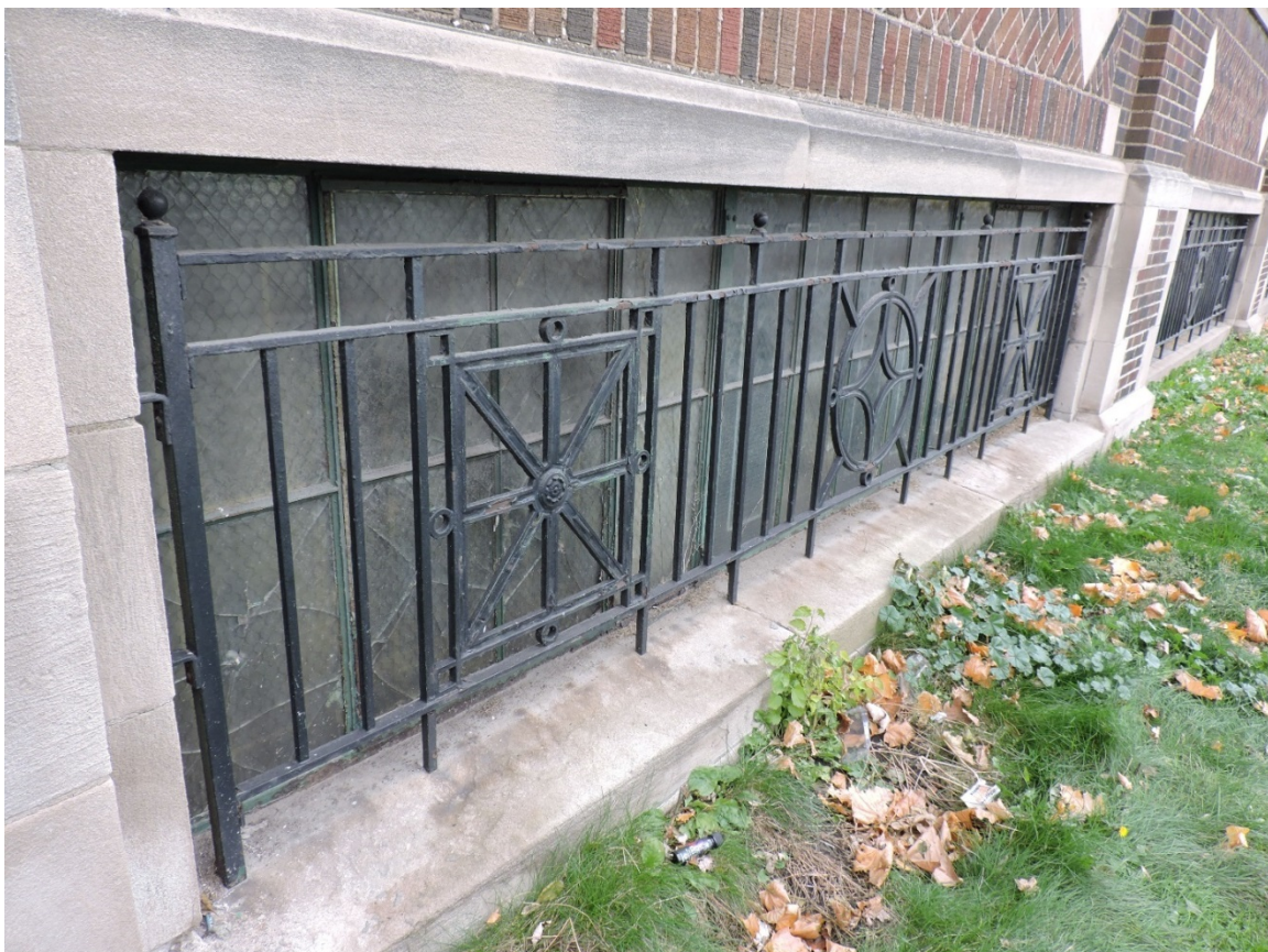
Figure 16 Barred basement windows on the front façade (AB, 2018).
