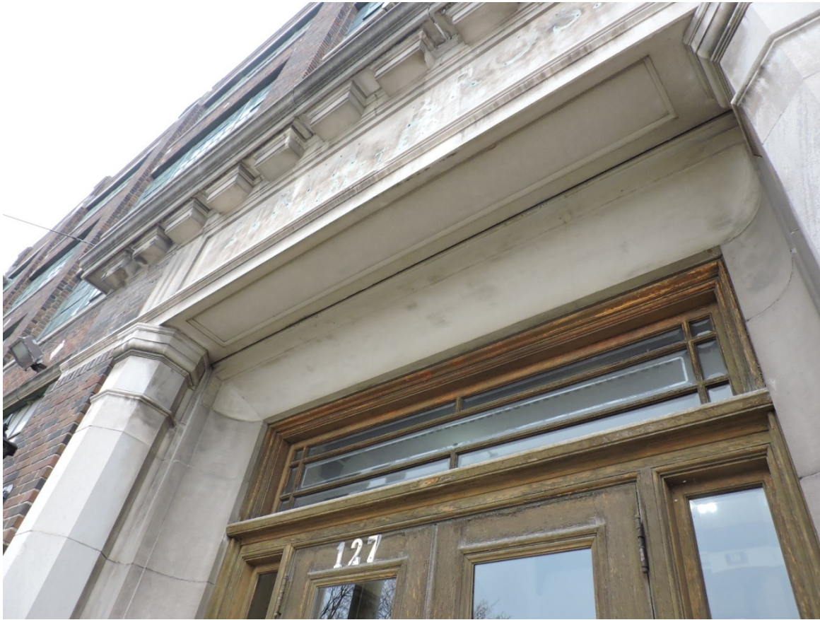
Figure 19 Front entranceway showing transom/lintel details and outline of erstwhile Firth Bros. brass lettering (AB, 2018).
