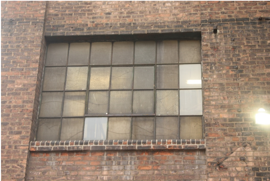
Figure 13 Original window of the old (west) section; south wall (ZH, 2018).
