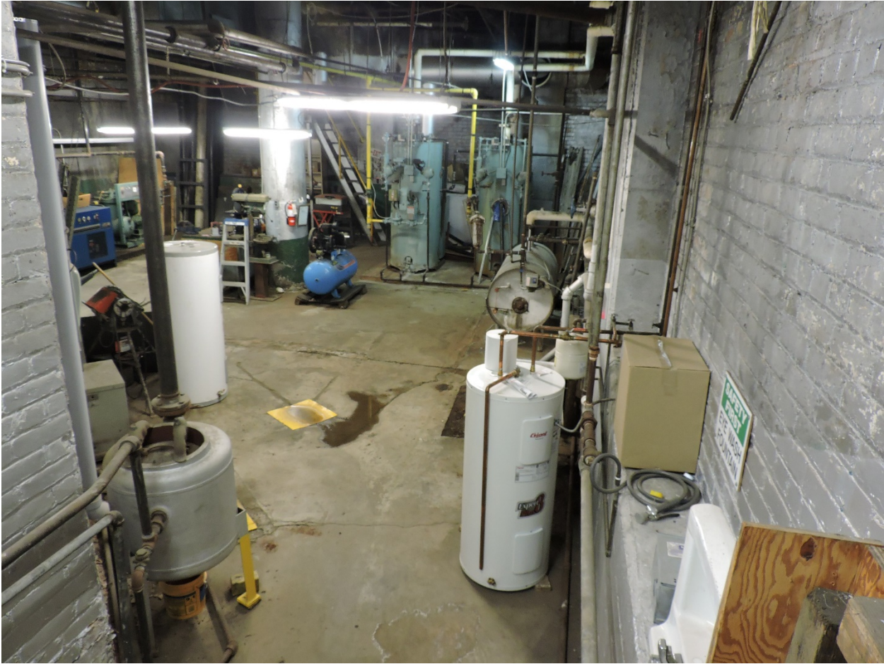
Figure 74 East section boiler room (AB, 2018).
