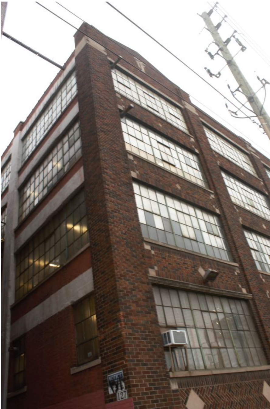
Figure 7 South corner of the east section/front façade of subject property (ZH, 2018).
