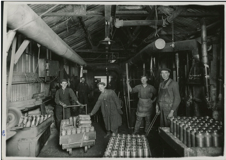
Figure 9: Stelco workers tending shell manufacturing in Hamilton. "Stelco workers pose proudly beside hundreds of shell cylinders made from molten steel" (Library and Archives Canada, 1940-, e01118373).
