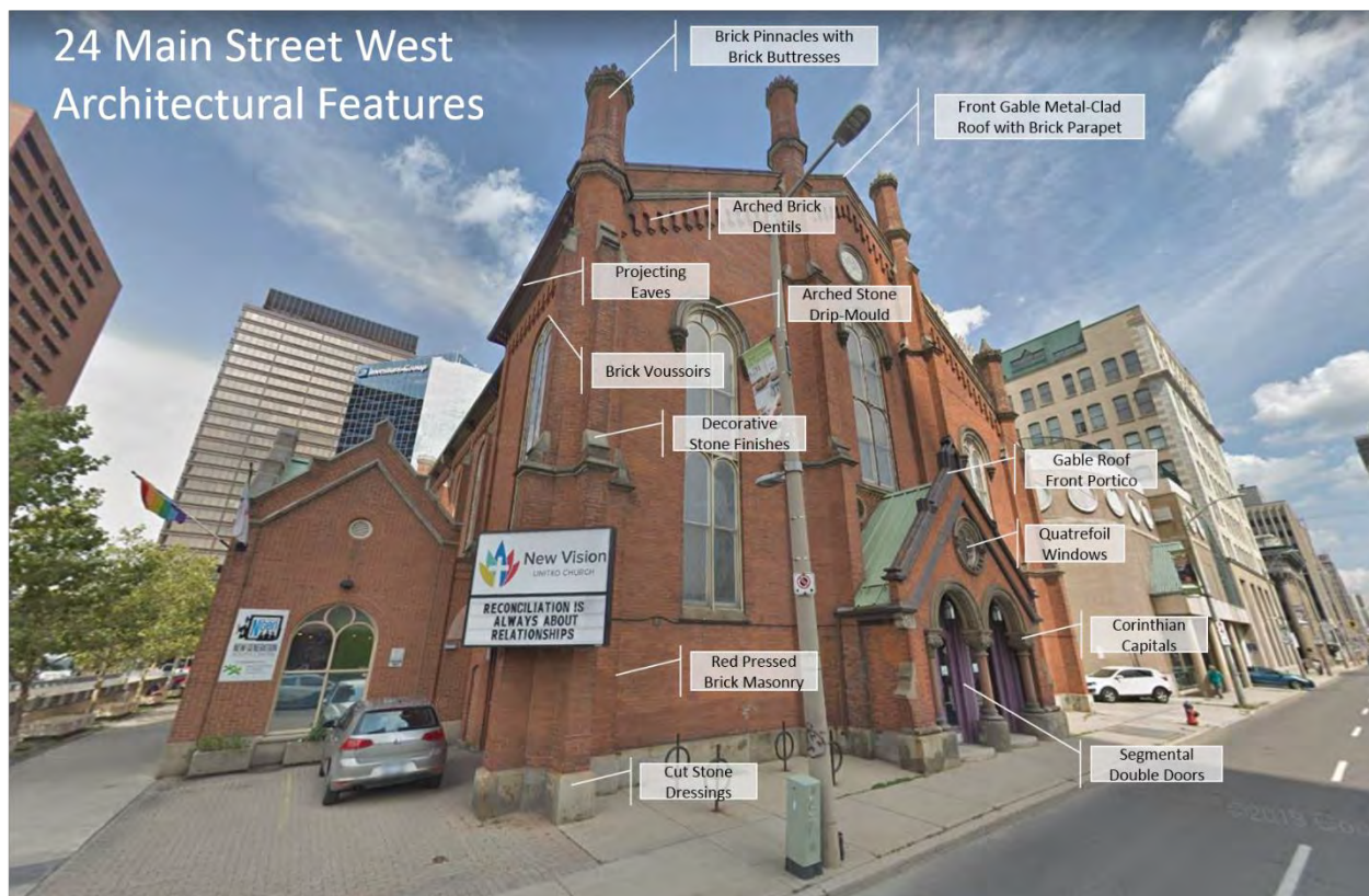
Image 8 – Visual of Significant Exterior Architectural Features. (Source: Google Maps).
