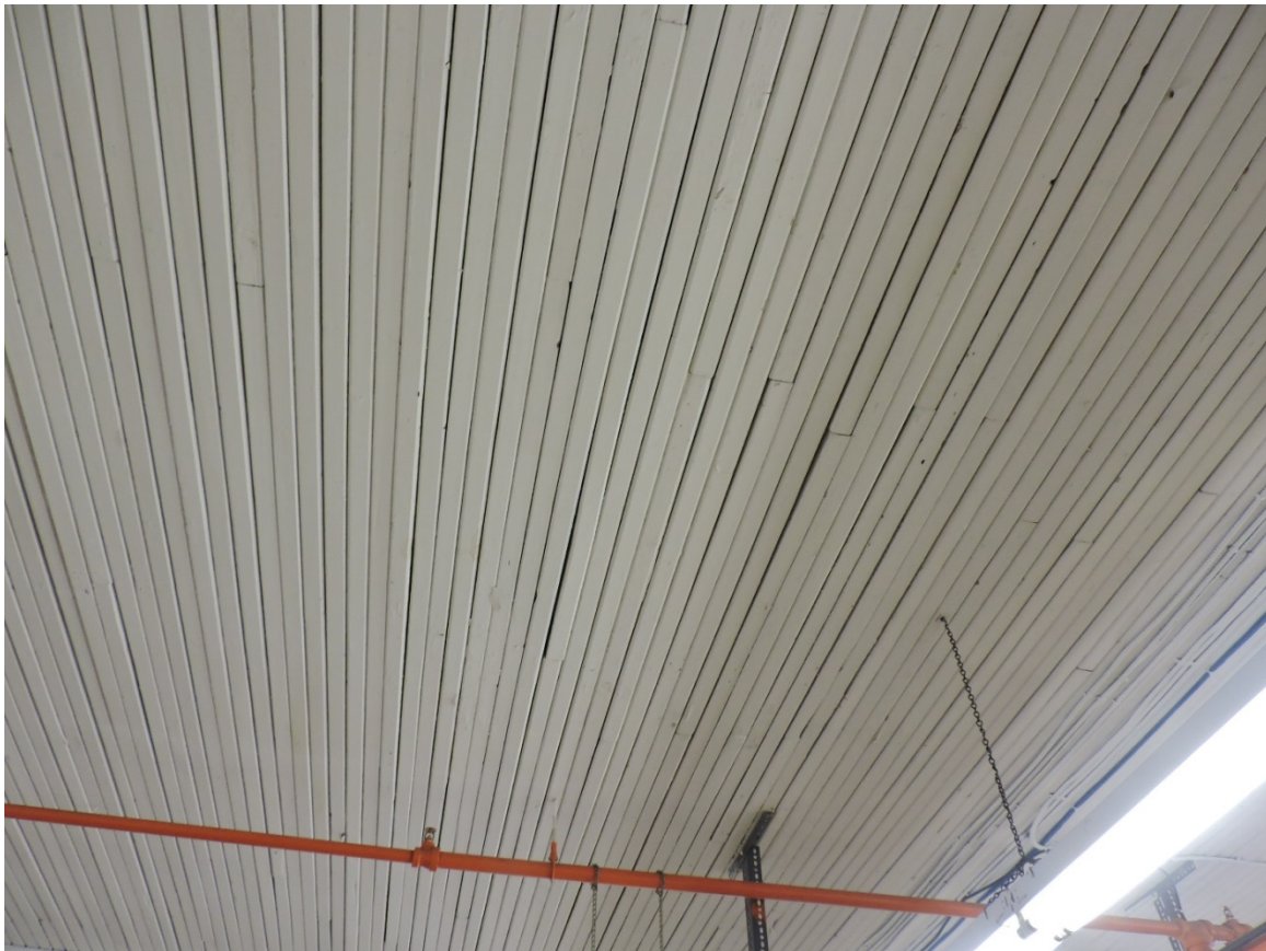
Figure 60 West section typical ceiling – wood planks painted white (AB, 2018).
