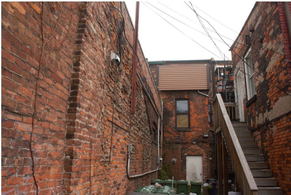
Figure 27 One-story level connecting shops to west section (ZH, 2018).
