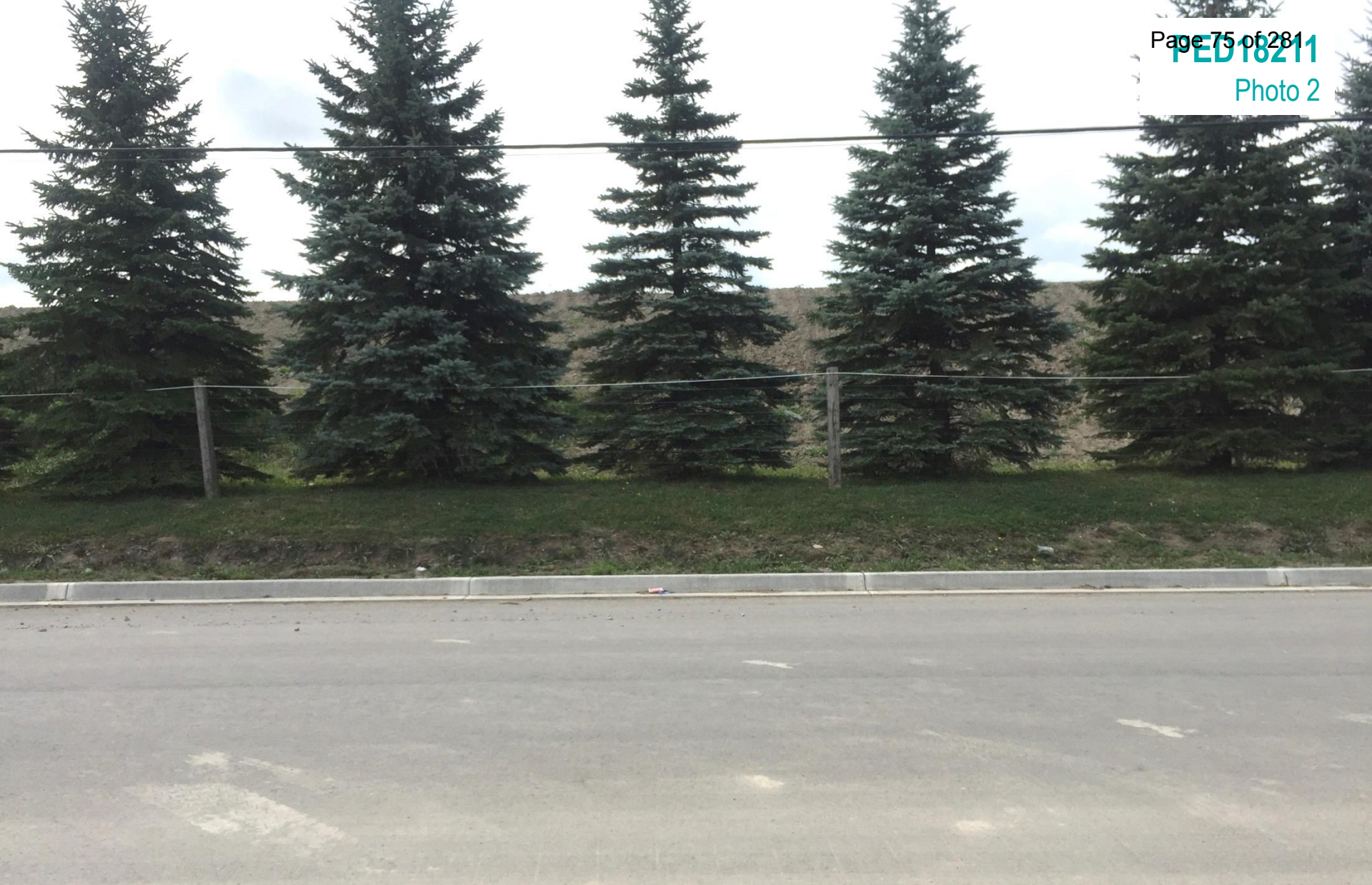
Looking south along Green Mountain Road West at Terrapure
