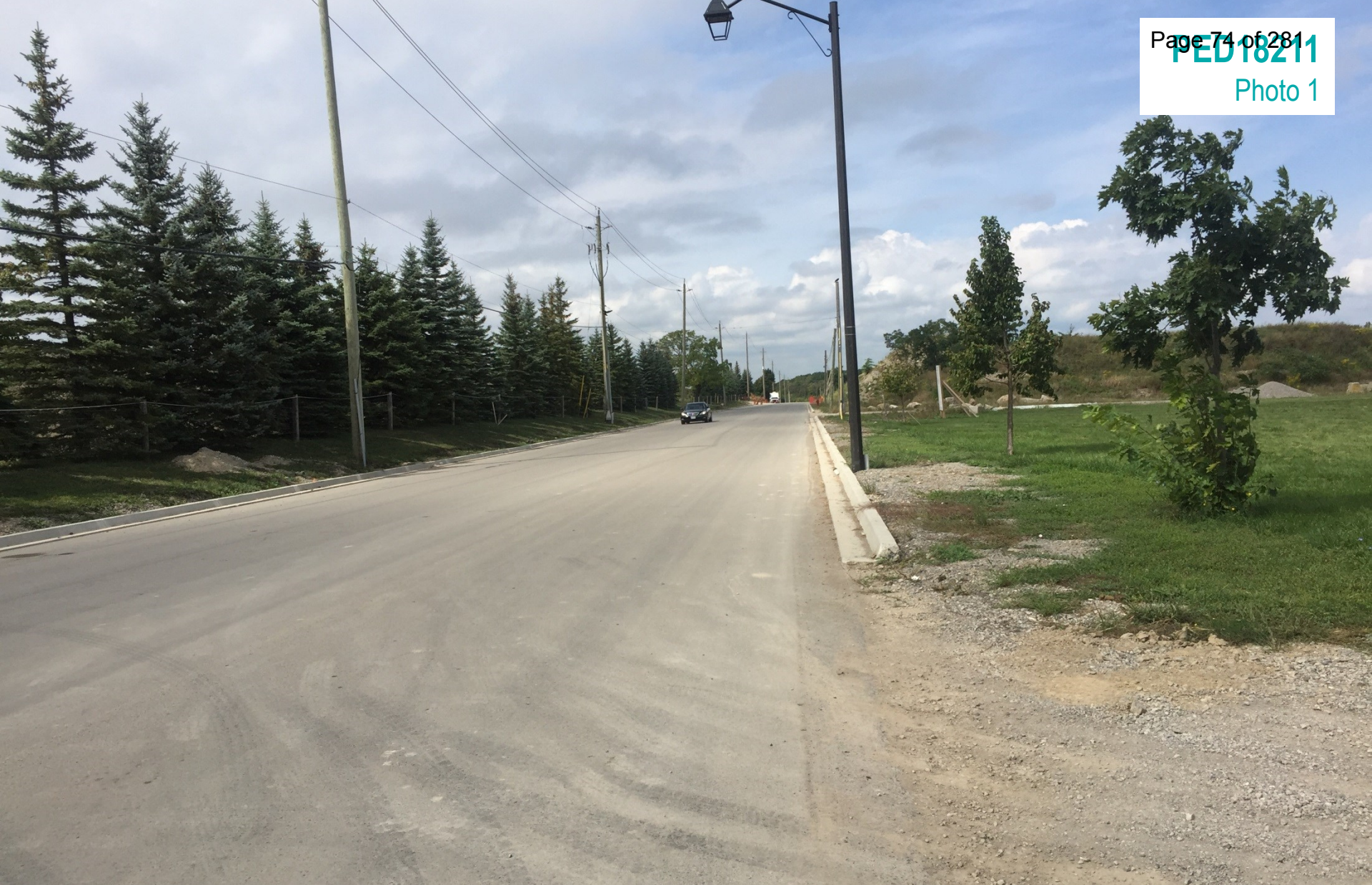
Looking west along Green Mountain Road West
