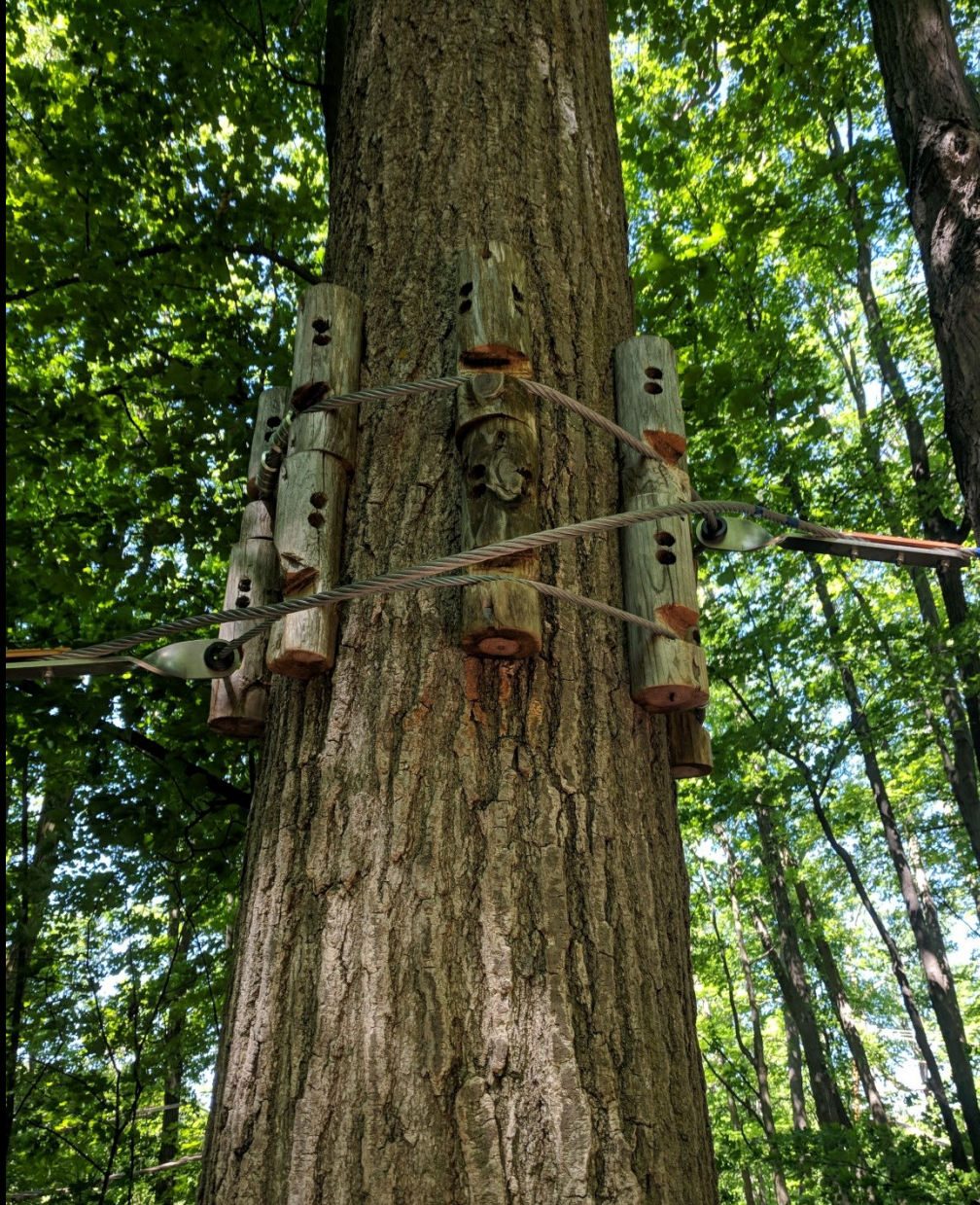
Trees are protected with "Tree Savers" Zip lines do not make contact with the tree (Brampton Location)
