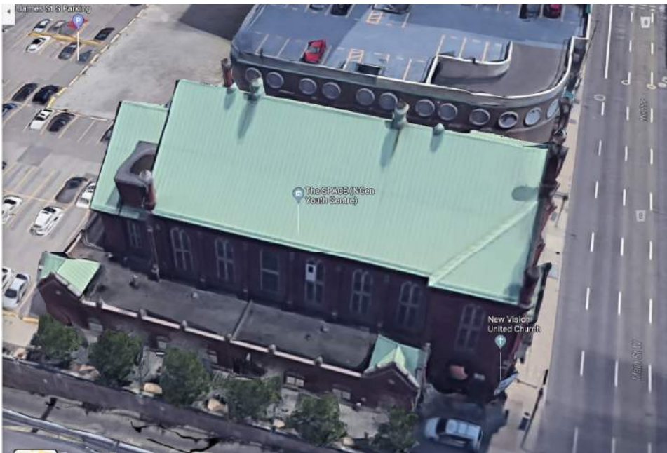
Figure 4.3 - Top: (source: Google maps) Aerial Photo
