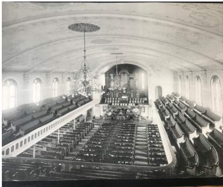
Figure 5.20 - (source - Hamilton Central Library) Dated c. 1899 - Interior view of auditorium from south east corner of upper gallery
