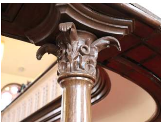
Figure 4.14 - Detail of Column supporting balcony
