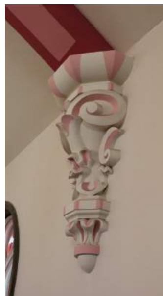
Figure 4.12 - Decorative painted plaster braket
