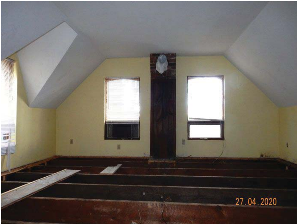
Figure 11: Interior Second Floor Room, Flooring Removed, 1389 Progreston Road
