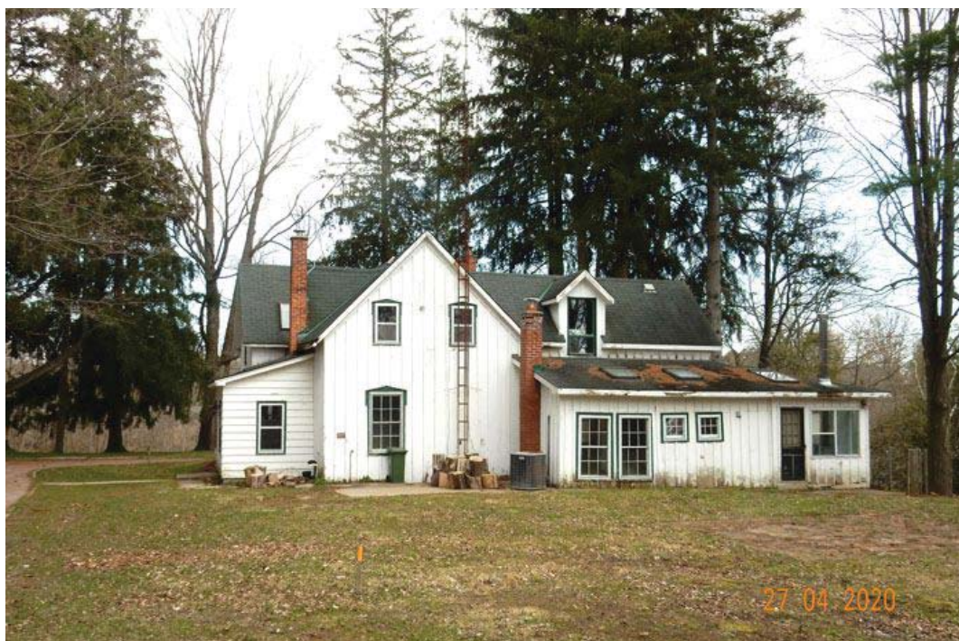
Figure 2: Rear Elevation, 1389 Progreston Road
