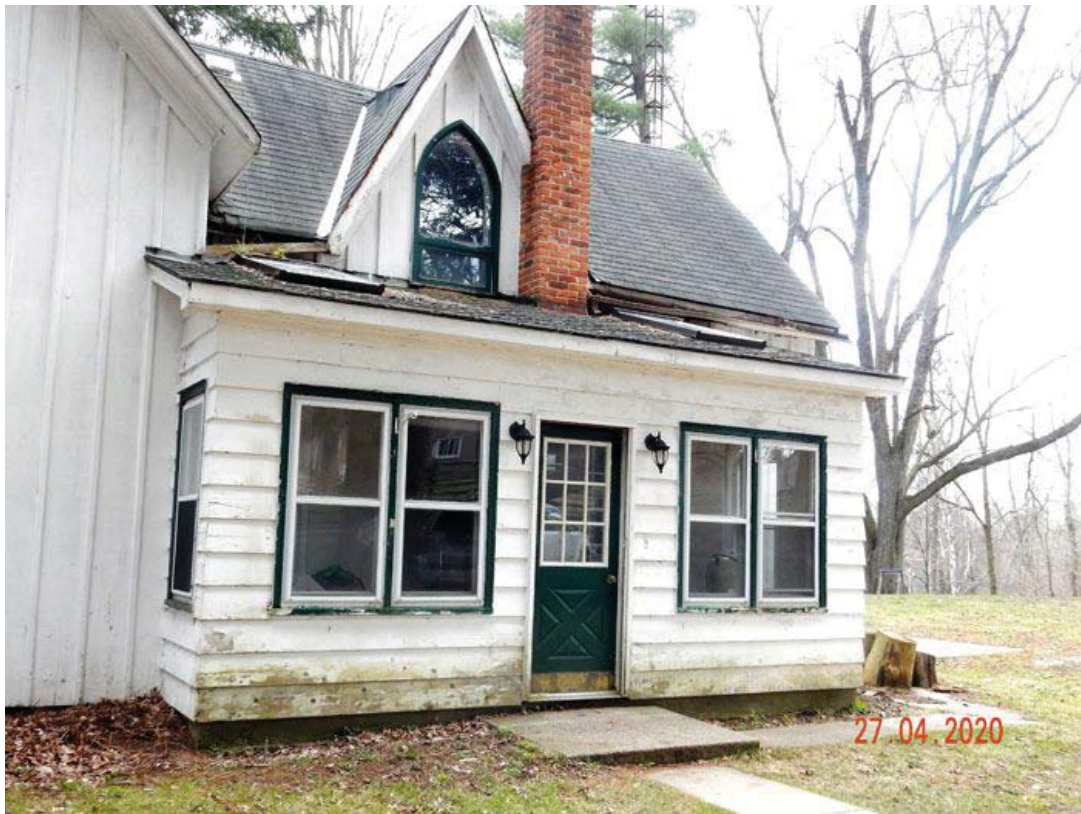
Figure 5: North Elevation, 1389 Progreston Road
