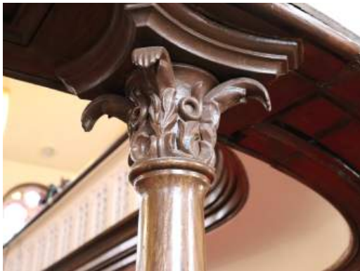
Figure 4.14 - Detail of Column supporting balcony
