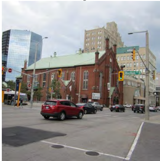
Brick Pinnacles & Buttresses
