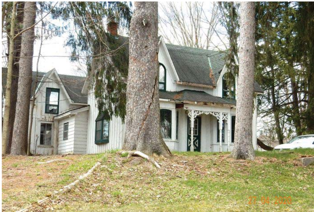
Figure 1: 1389 Progreston Road, Facade from Progreston Road
