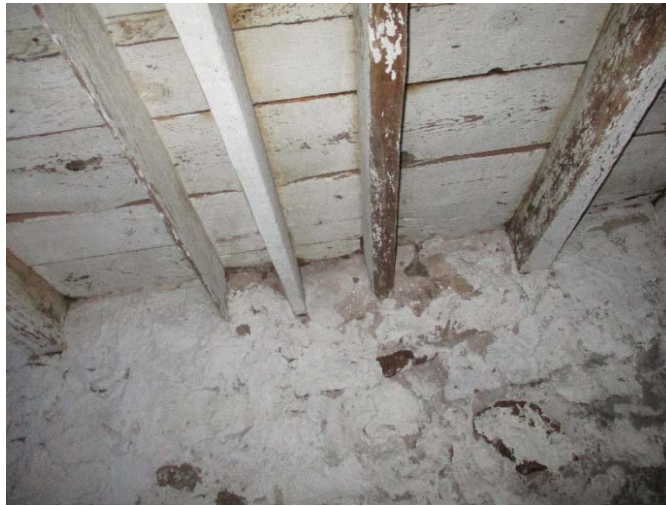
Randomly sized and spaced circular-sawn floor joists
