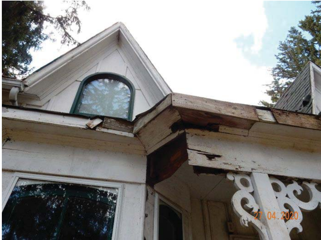
Figure 7: Corner of Porch and Gable Above, 1389 Progreston Road
