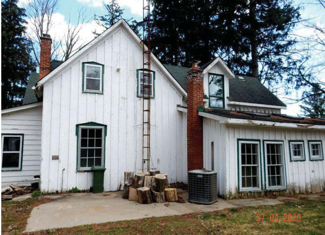
Figure 4: Rear Elevation, 1389 Progreston Road
