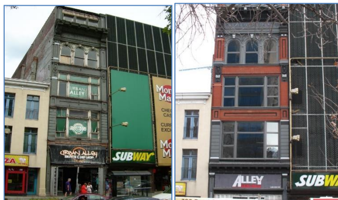
11 King Street East, Hamilton (before and after)
