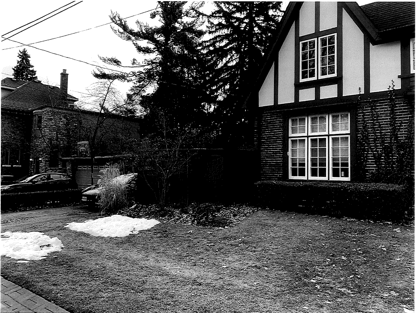
66 Oak Knoll Drive showing existing deck and fence.
