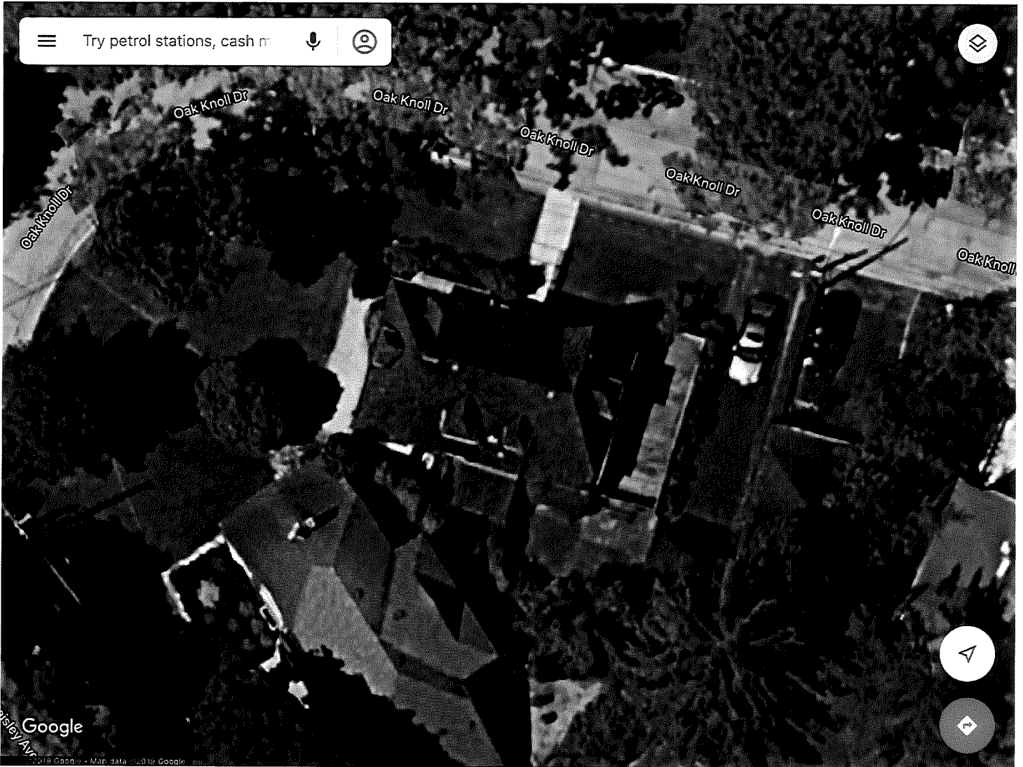
airial view of 66 Oak Knoll Drive showing existing deck
