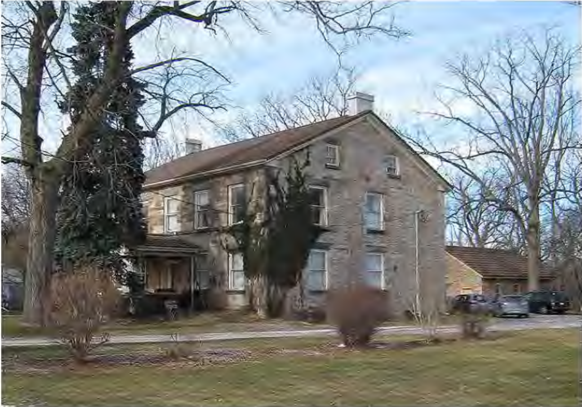
Appendix G – Looking northeast at the home with part of stone stable in view (courtesy Brian Kowalewicz).
