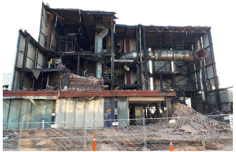
Figure 2: Demolition of Existing Facility (2018)
