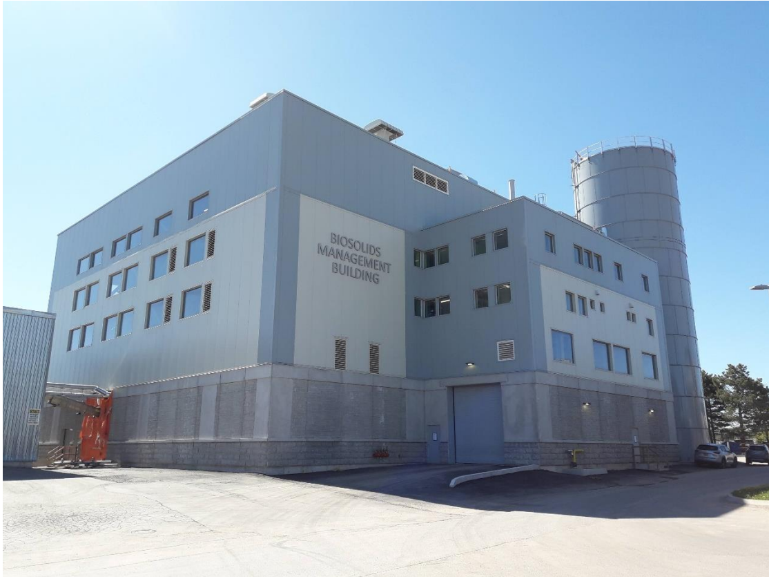
Figure 10: Finished Facility Exterior, North-West Elevation (2020)
