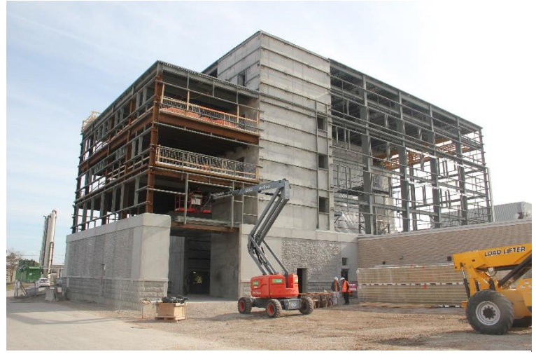
Figure 4: Structural Steel Construction (2019)
