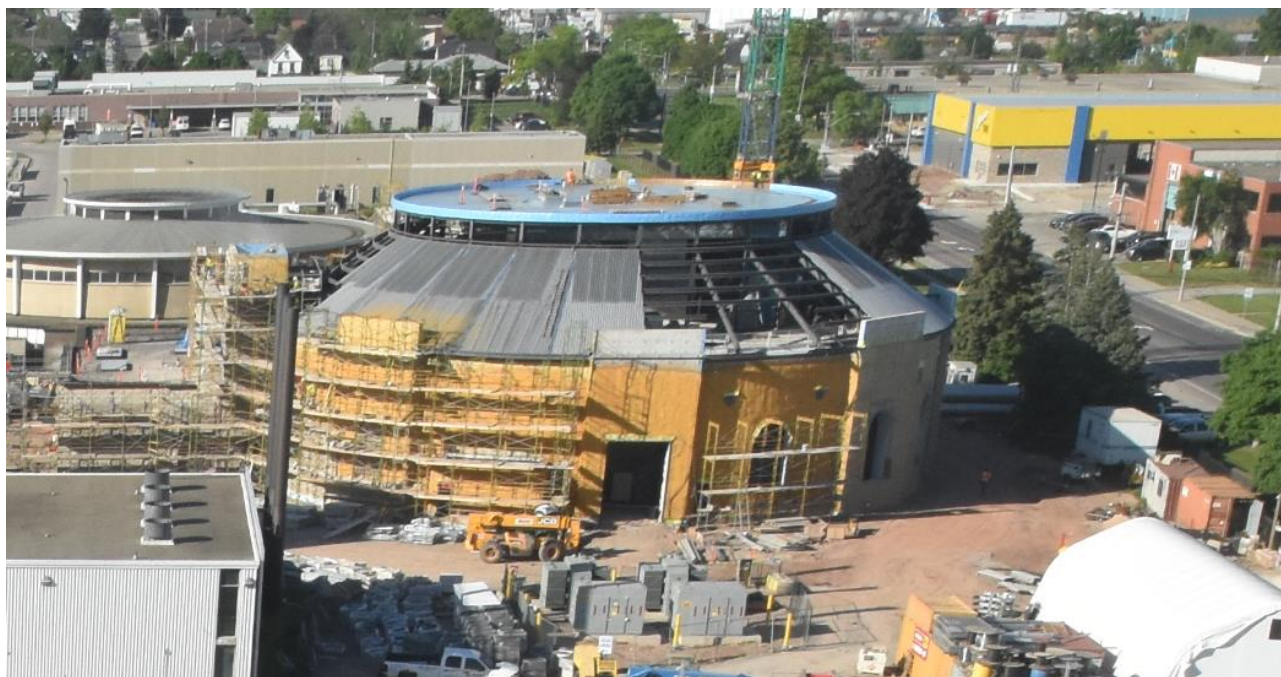
Figure 2: New Main Pumping Station
