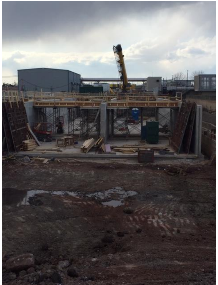
Figure 9: South Aeration Plant Expansion Construction
