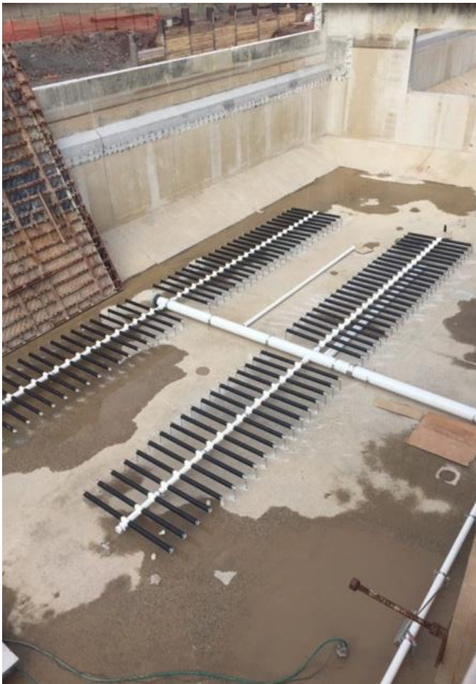
Figure 4: South Aeration Plant Expansion Construction
