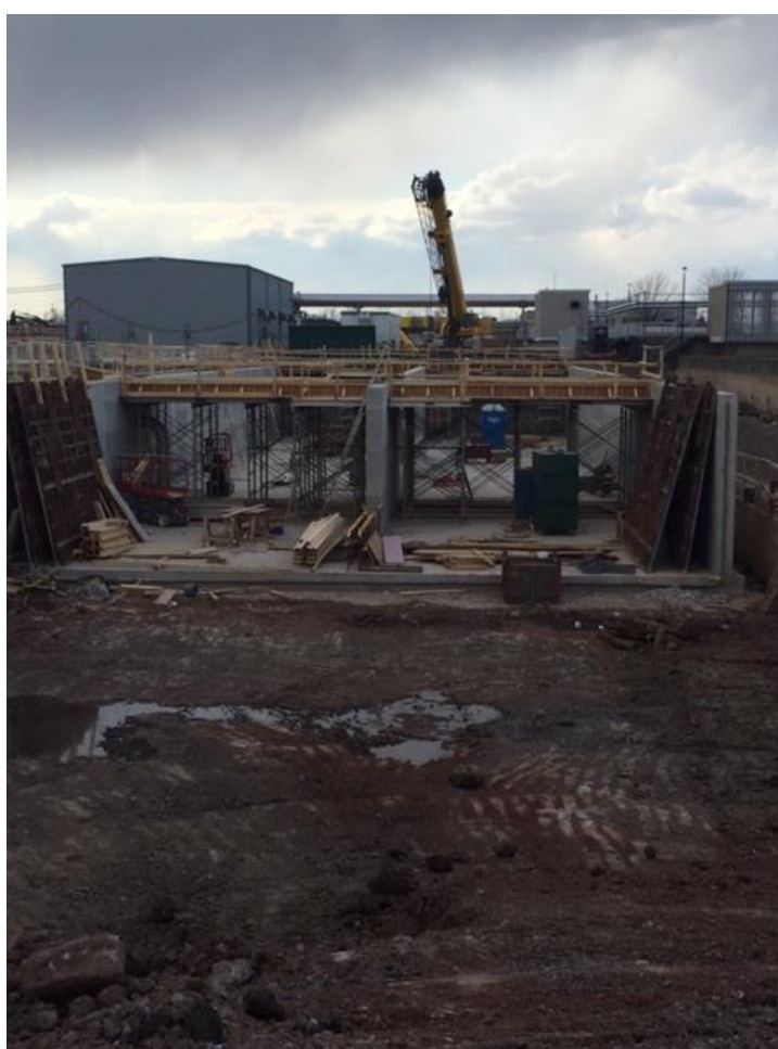
Figure 9: South Aeration Plant Expansion Construction
