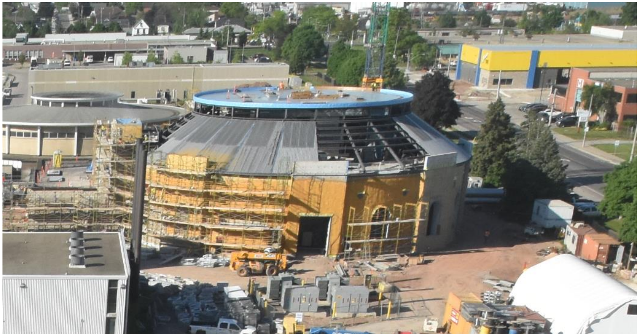
Figure 2: New Main Pumping Station
