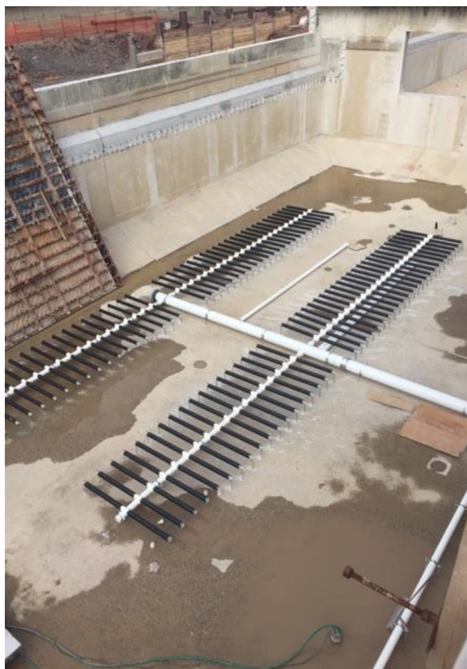
Figure 4: South Aeration Plant Expansion Construction
