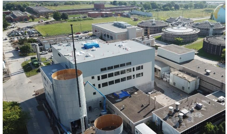
Figure 6: Dry Pellet Storage Silo Construction (2019)
