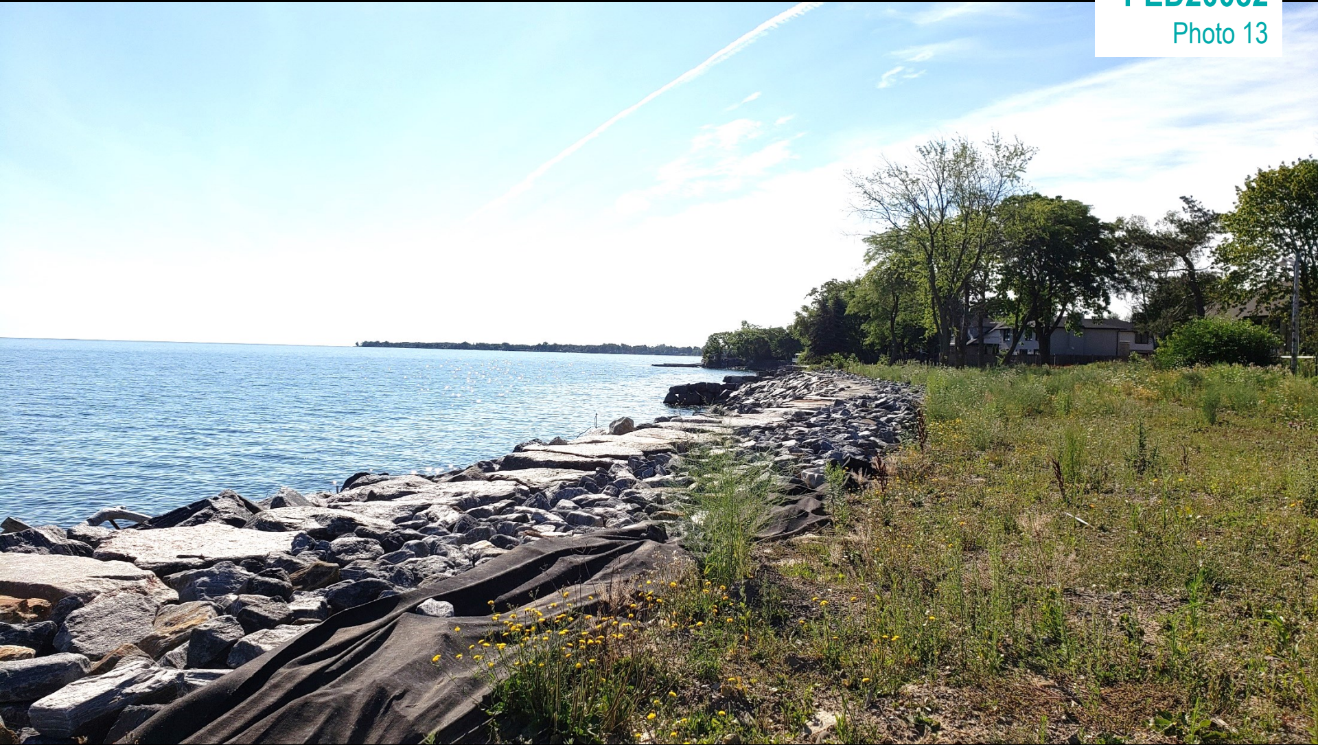
View to the east along the shoreline retaining wall
