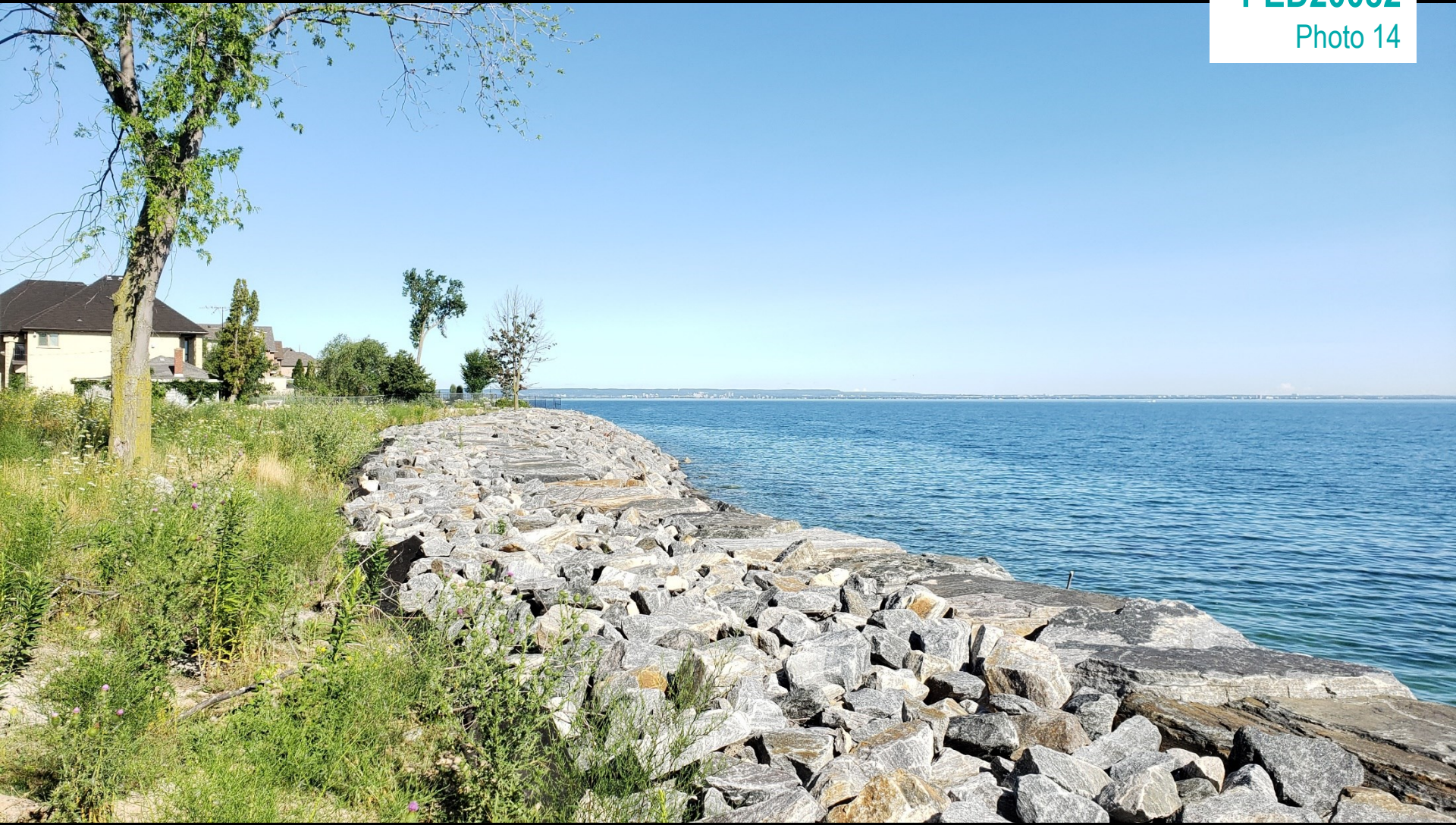
View to the west along the shoreline retaining wall
