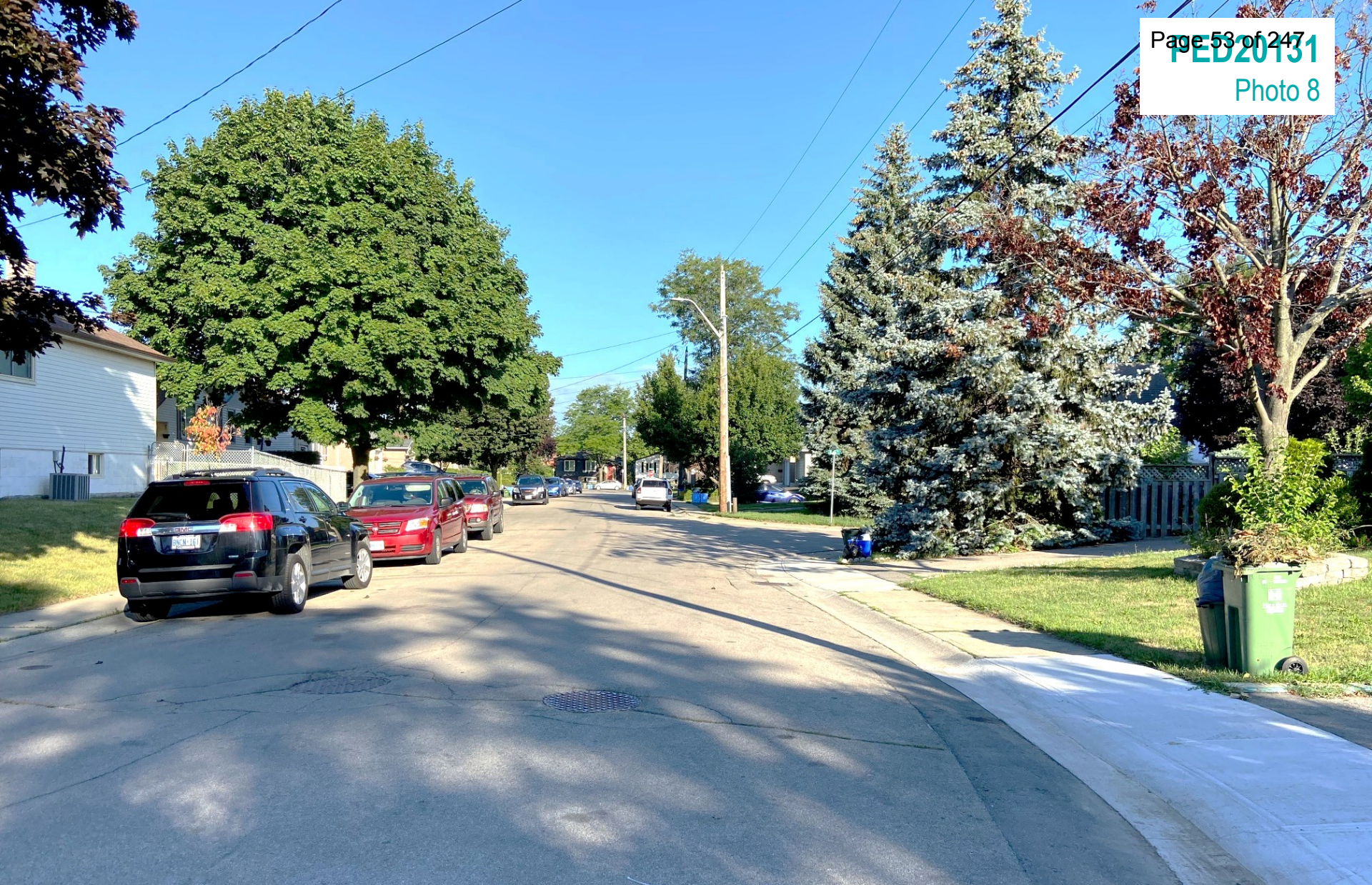
1406 Upper Gage - Along Elmore Drive Facing West
