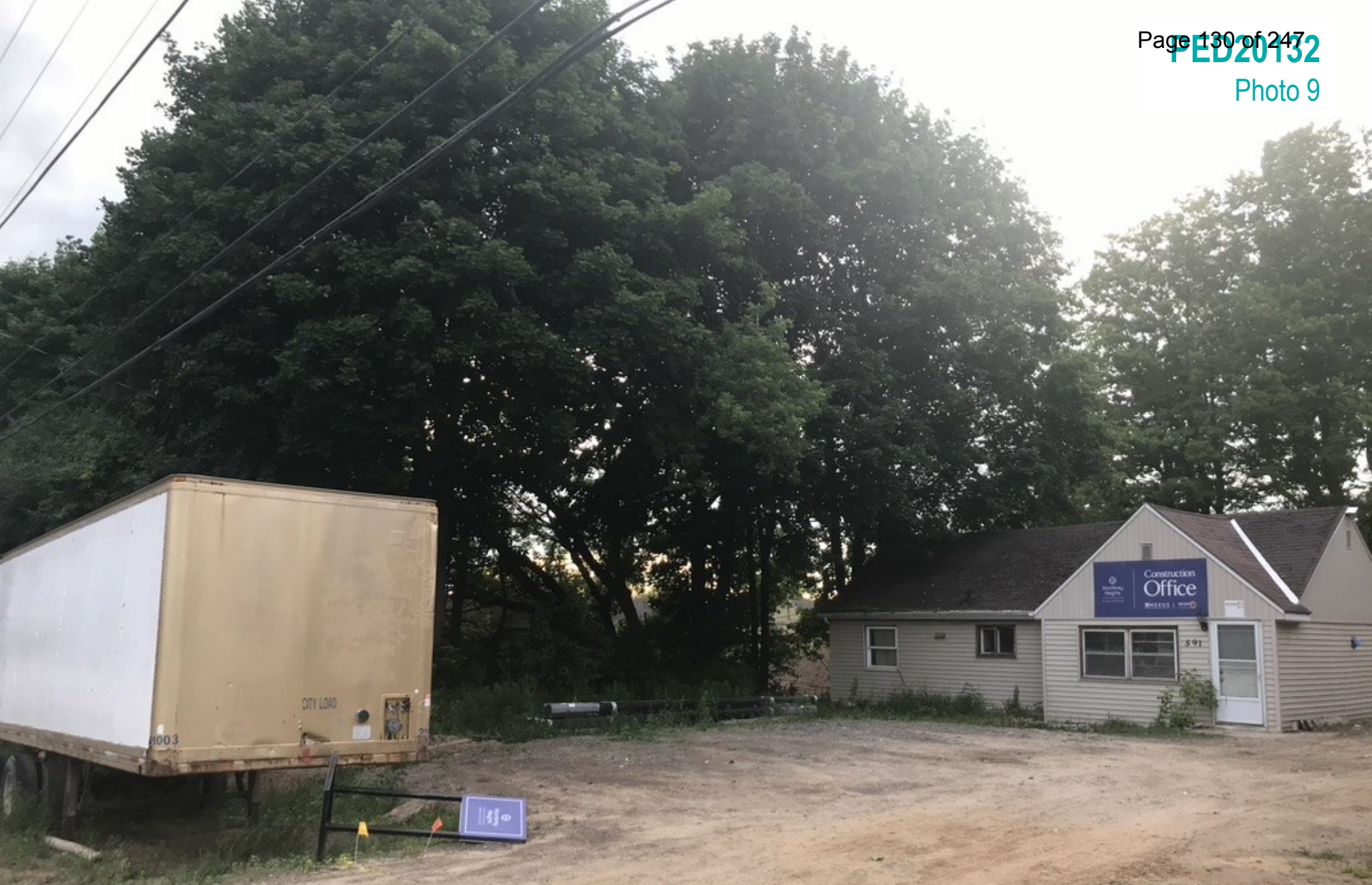
Southerly portion of subject lands from Garner Road West – existing dwelling
