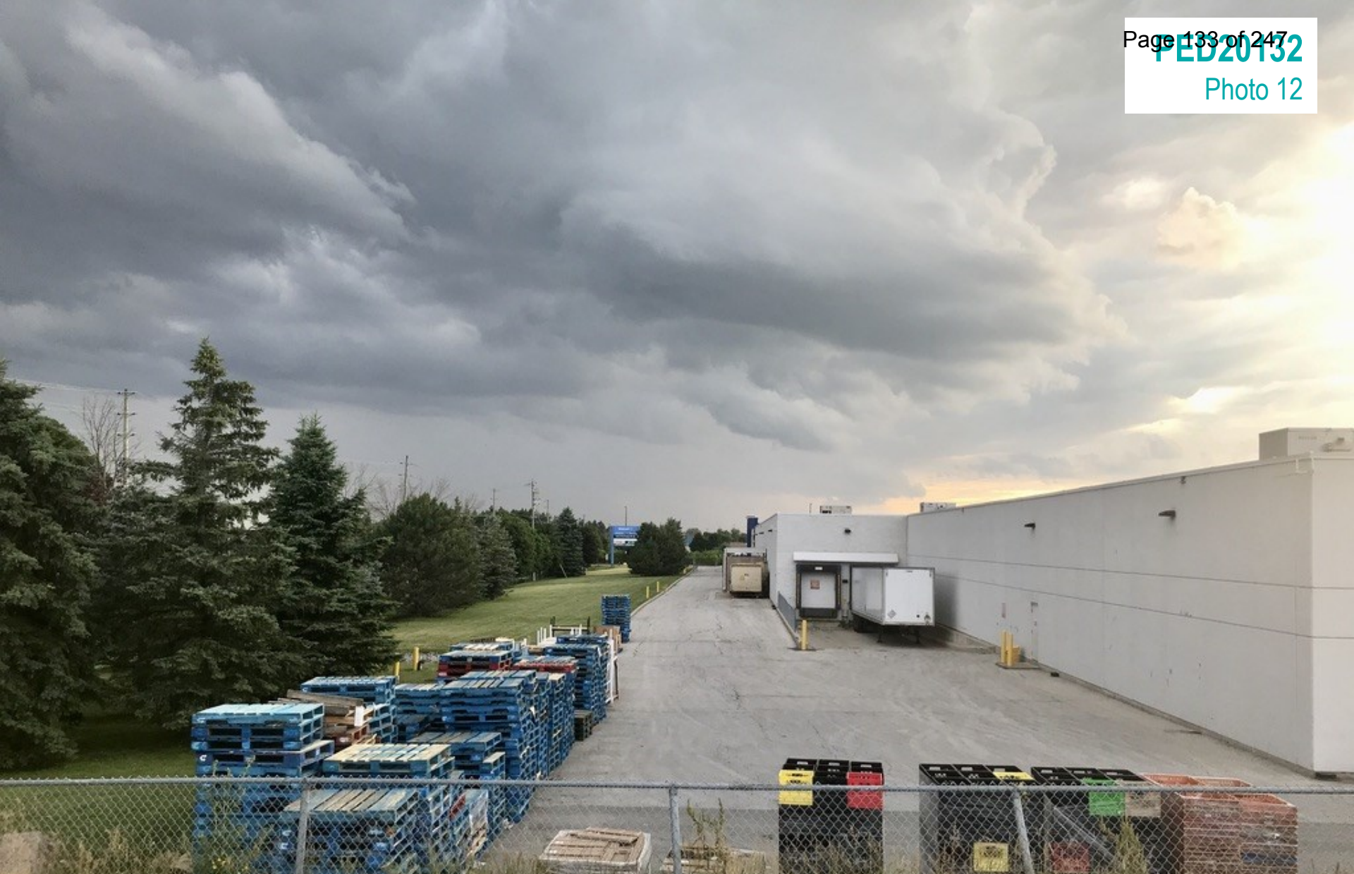
View of Walmart loading docks
