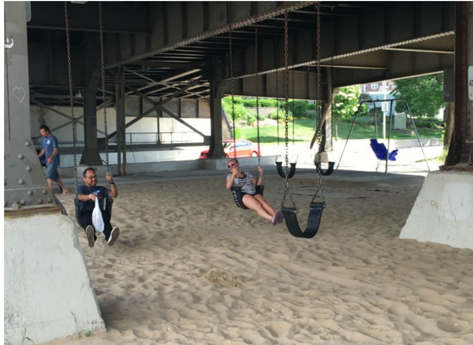
Holton Street Bridge Swings (USA)
