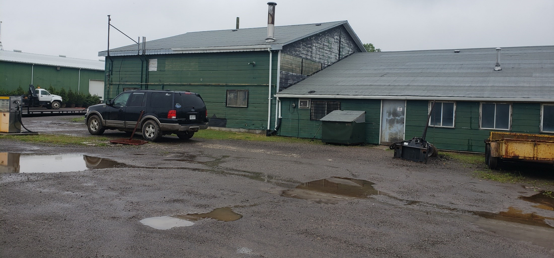
Building to be demolished
