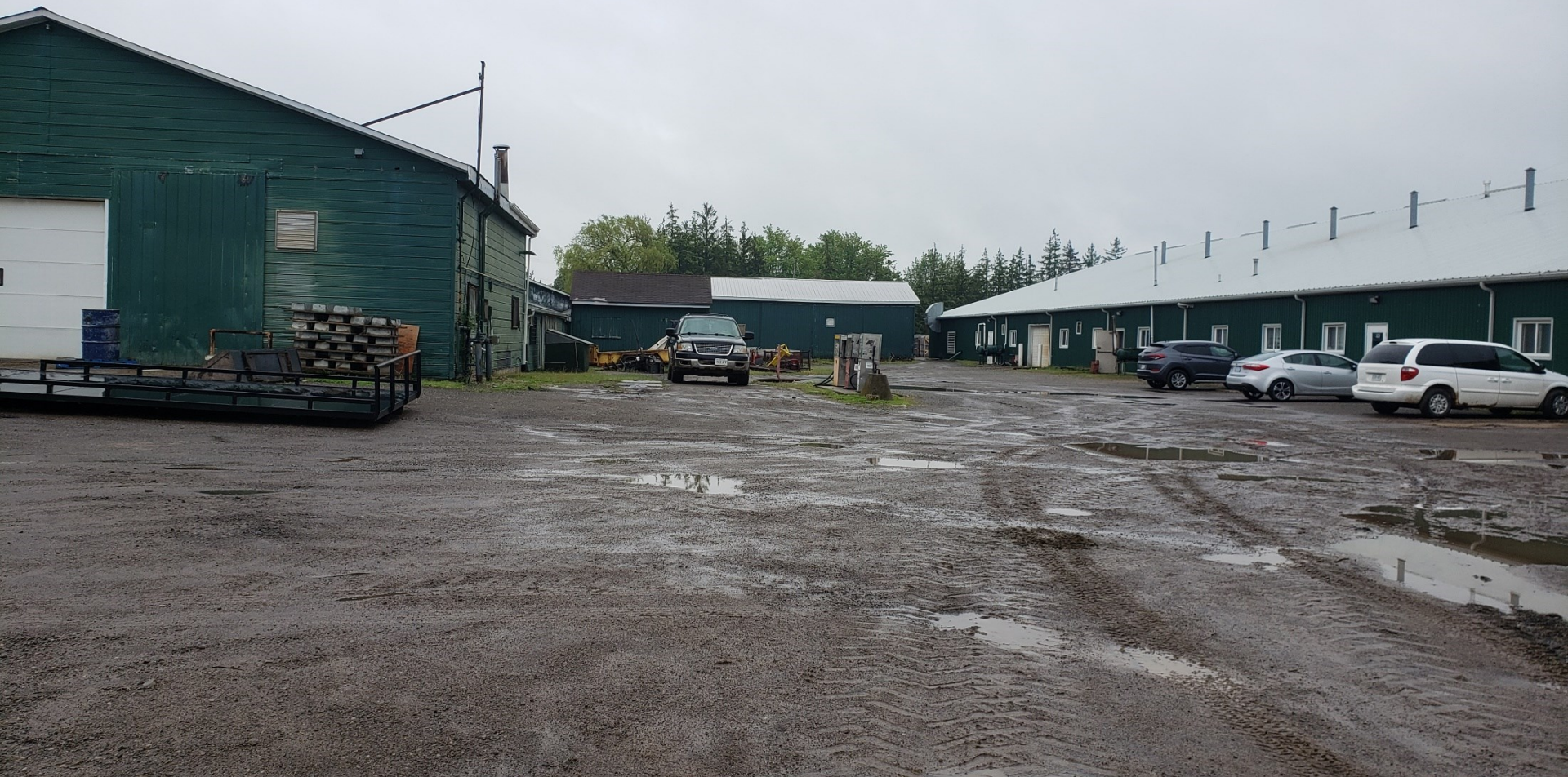
Existing Wire Basket Building
