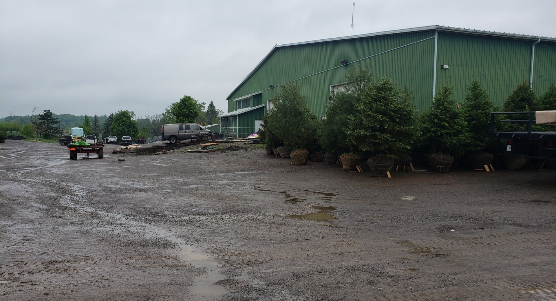
Storage Building for Nursery
