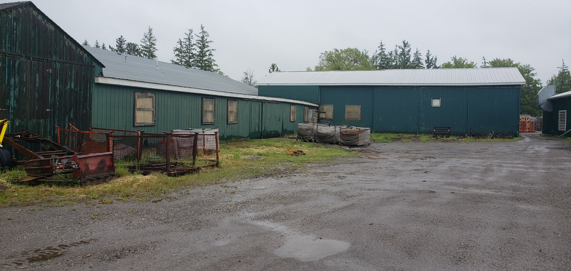
Building to be demolished
