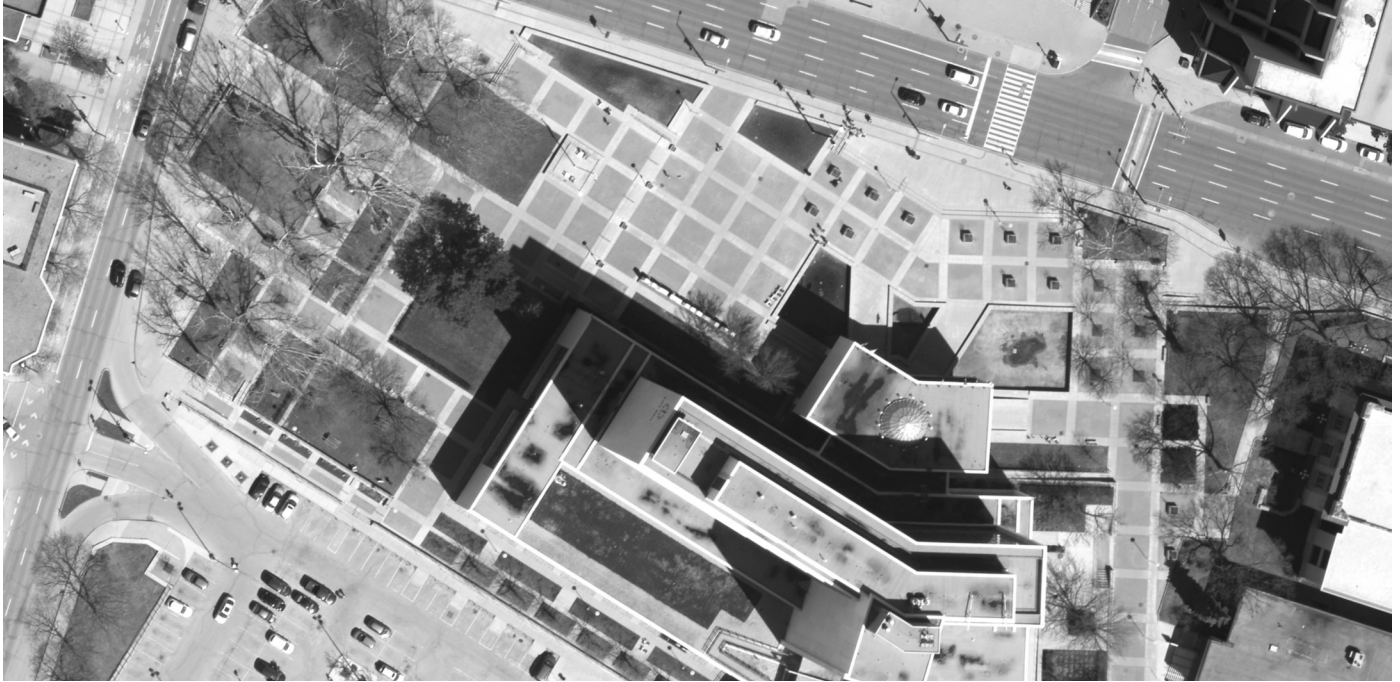
Figure 1: City Hall site
