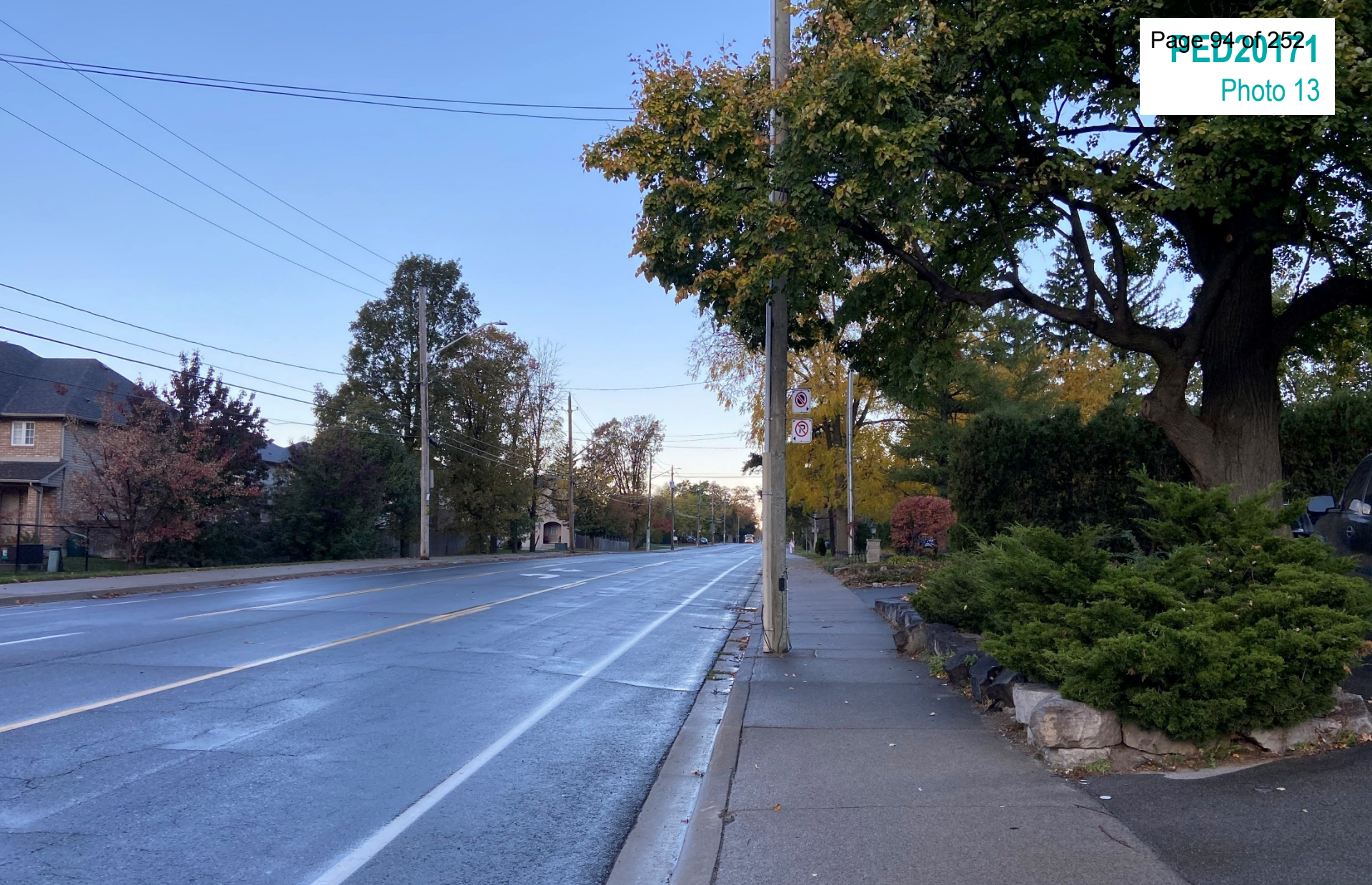
Stone Church Road West (looking west)
