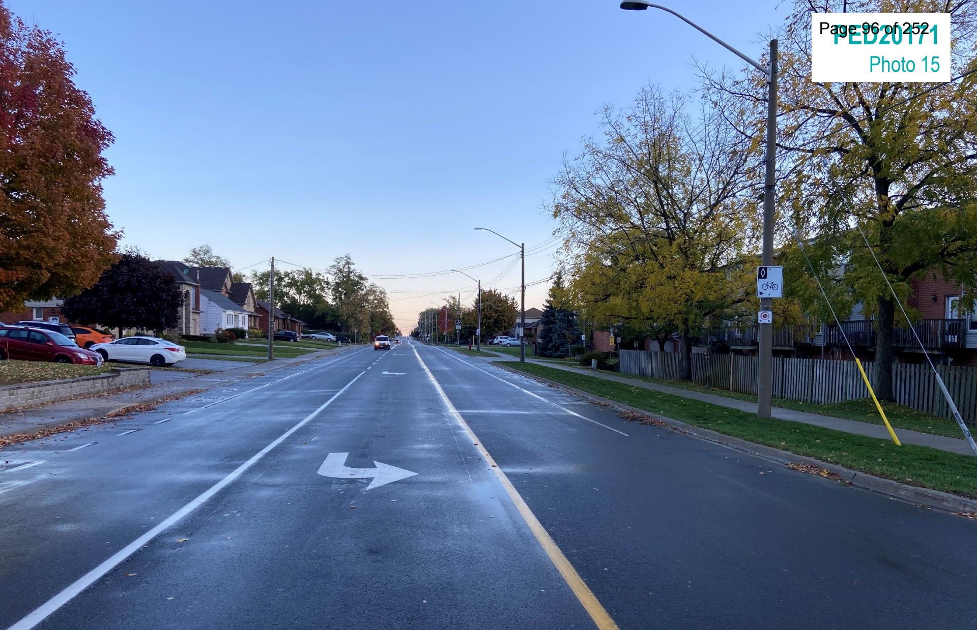
West 5 th Street (looking north)
