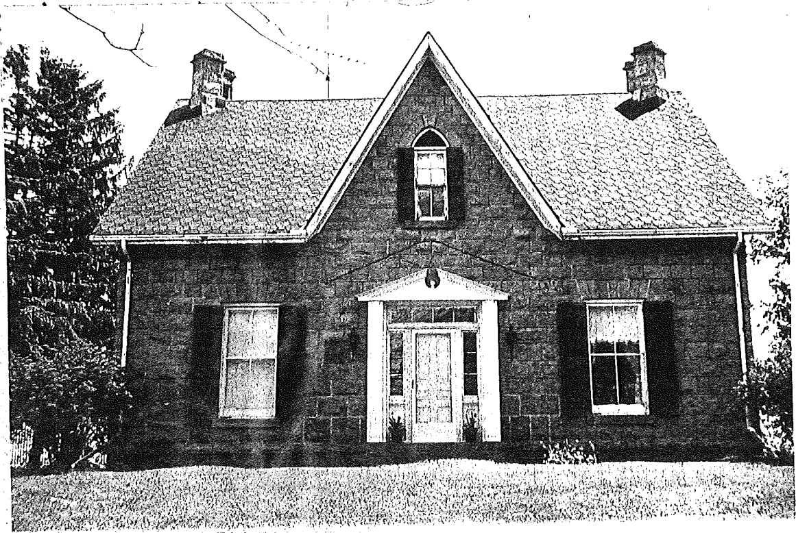
WEST (FRONT) VIEW ↑
