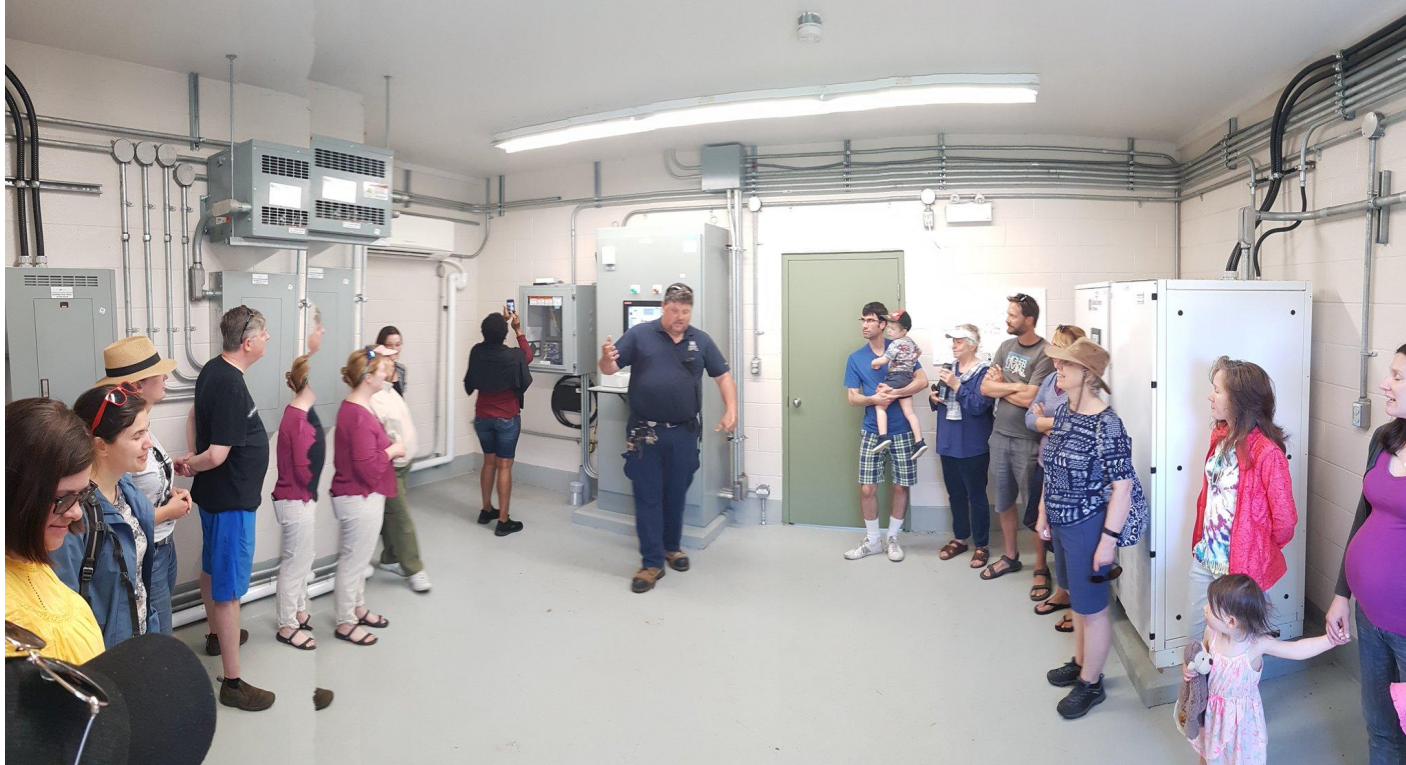
Neighbourhood Environment Walk tour of CSO control station provided by City staff.
