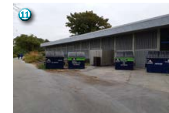
11 Garbage pick-up area is unsightly and has no buffer from the waterfront trail users.
