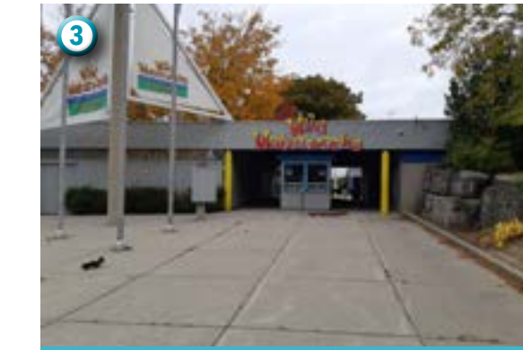
3 Dated signage, poorly defined entrance. Dark, cramped entry with only two ticket booths.
