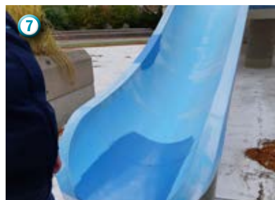
7 The slides and pool surfacing in Squirt Works is visibly degrading.
