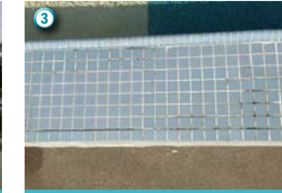
3 Wave pool surfacing and tile is degrading, potentially leading to sharp debris in the wave pool, posing a safety risk.
