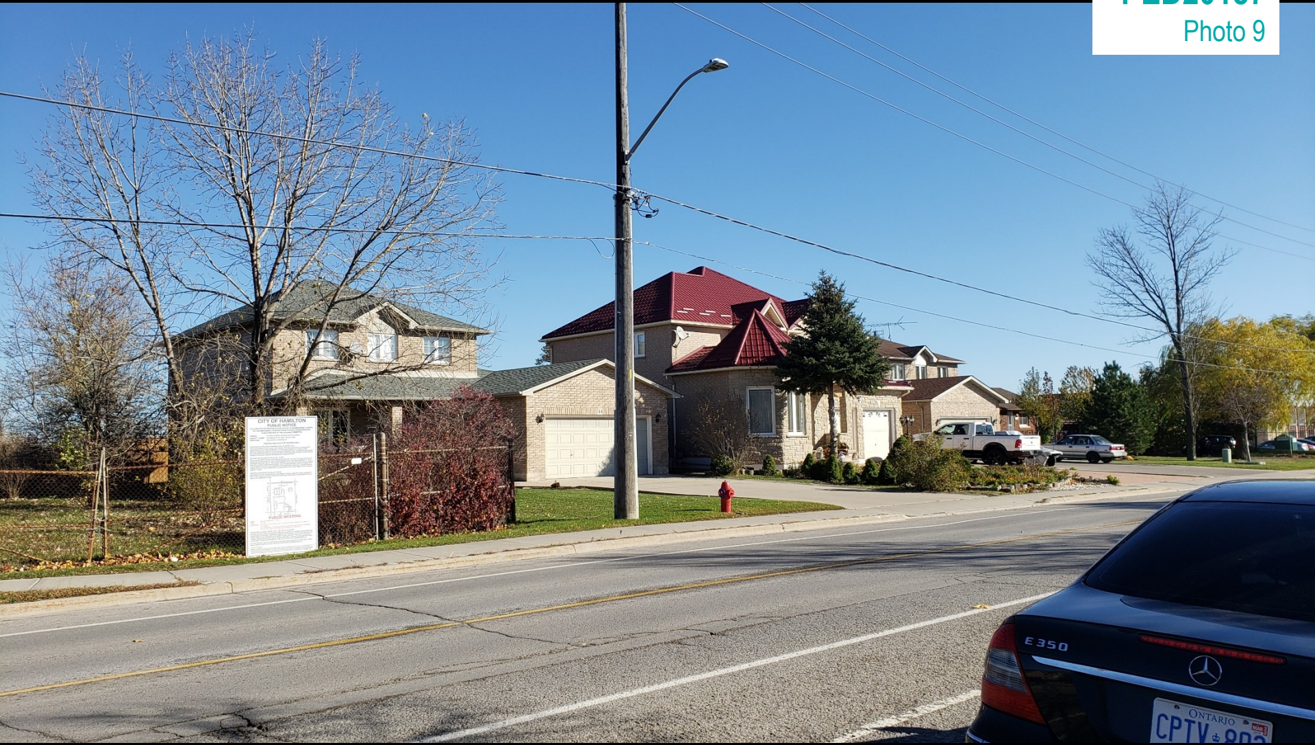
Single detached dwellings along Highland Road West to the east
