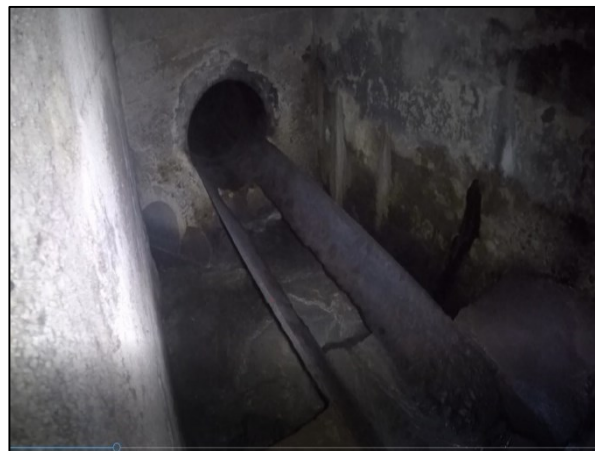
Regulator repair – Campbell Ave/Fraser Ave.
