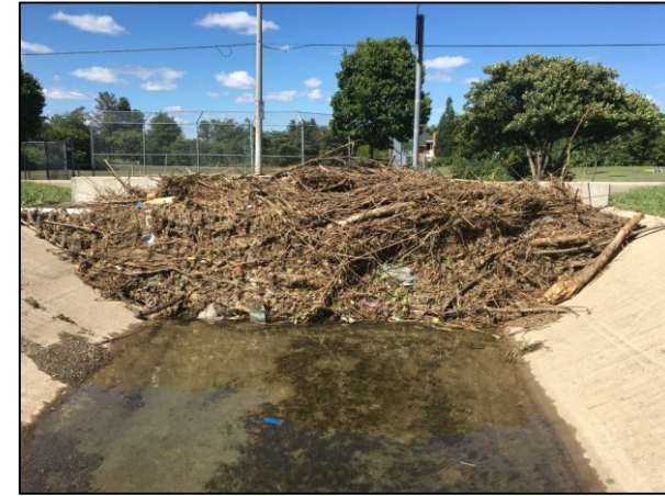
Sanatorium SW inlet / outlet – Rice Ave. & Sanatorium
