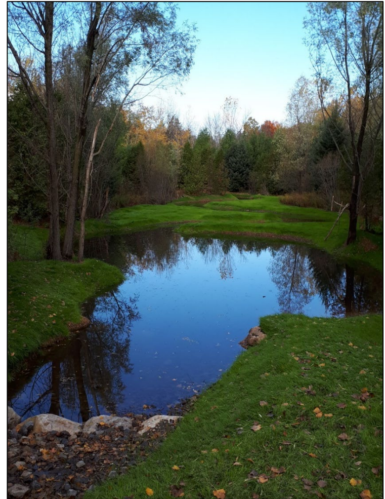
Stormwater Management Pond - Carlisle
